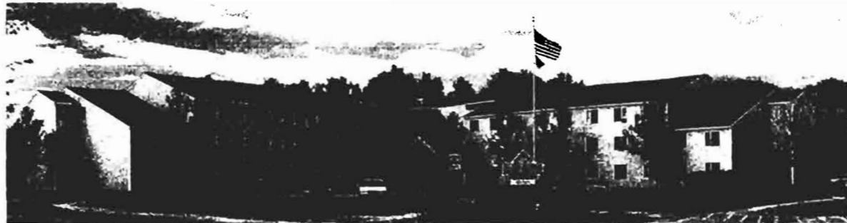
Mill Brook Estates. 100 units senior rental
