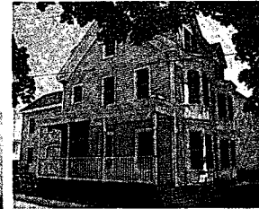
783 Main Street, complete renovation of historic Main Street property
