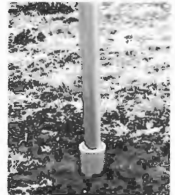
Footing plate Installed 3" Below Ground
