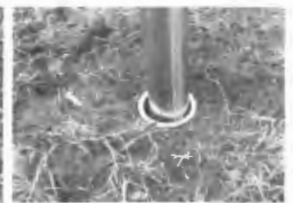
Match-Drill A Hole In The Post Through The Pre-Drilled Hole In The Sleeve And Secure With A Bolt
