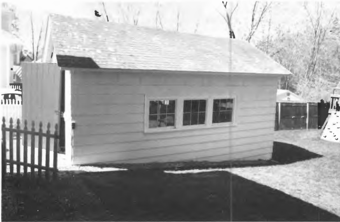
Front of garage, right side of garage, gate is attached to back left corner of house.
