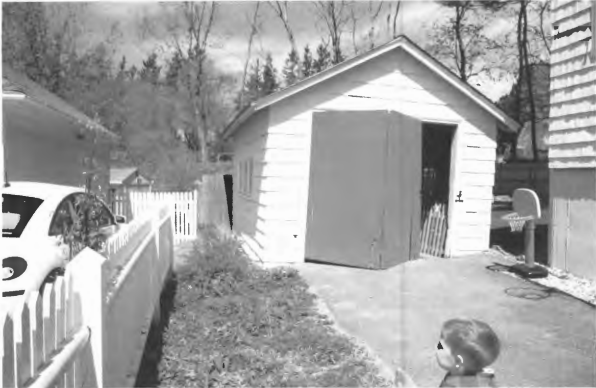
Left side of garage, back left corner of house.
