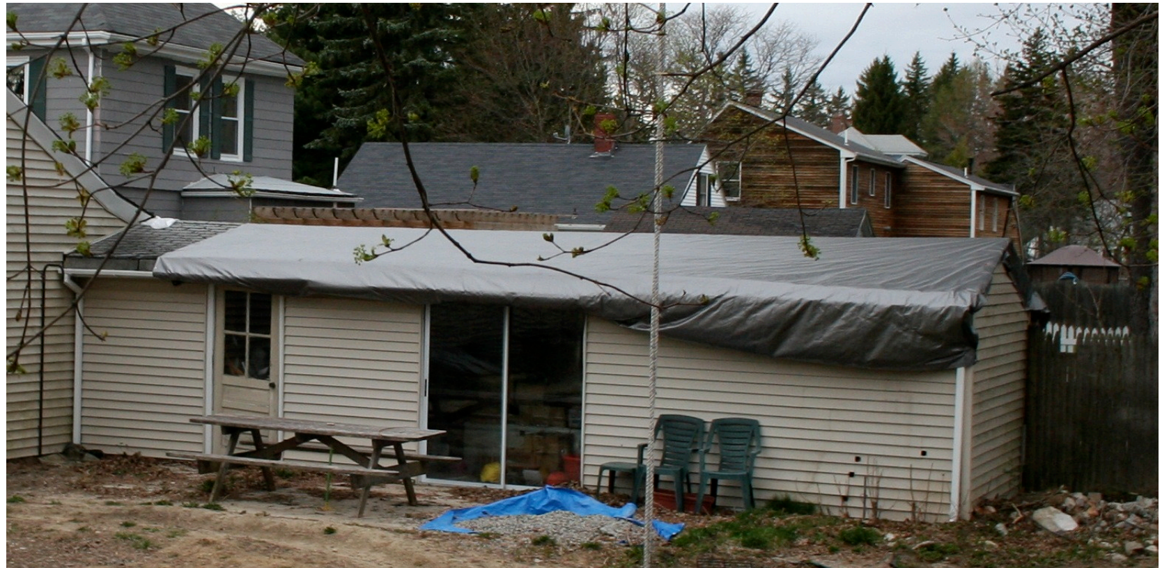
EXISTING SHED: SIDE VIEW
