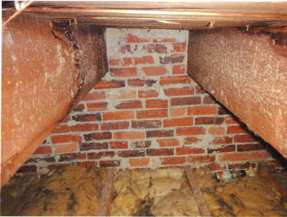
Photo 3: Sample photo showing the existing roof construction below the FRP chimney.
