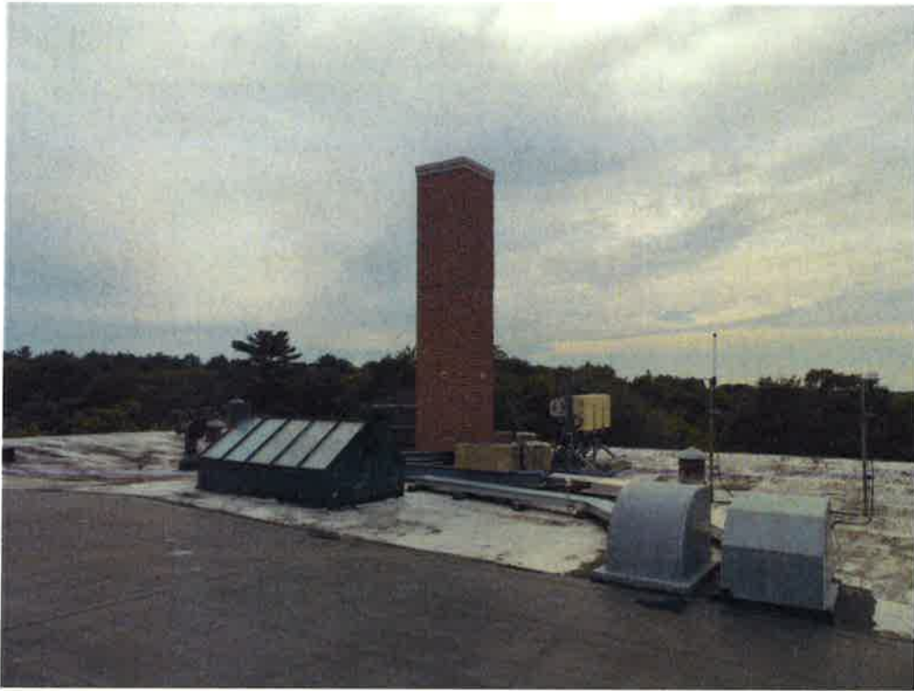
Photo 1: Sample photo showing the existing ballasted FRP chimney.
