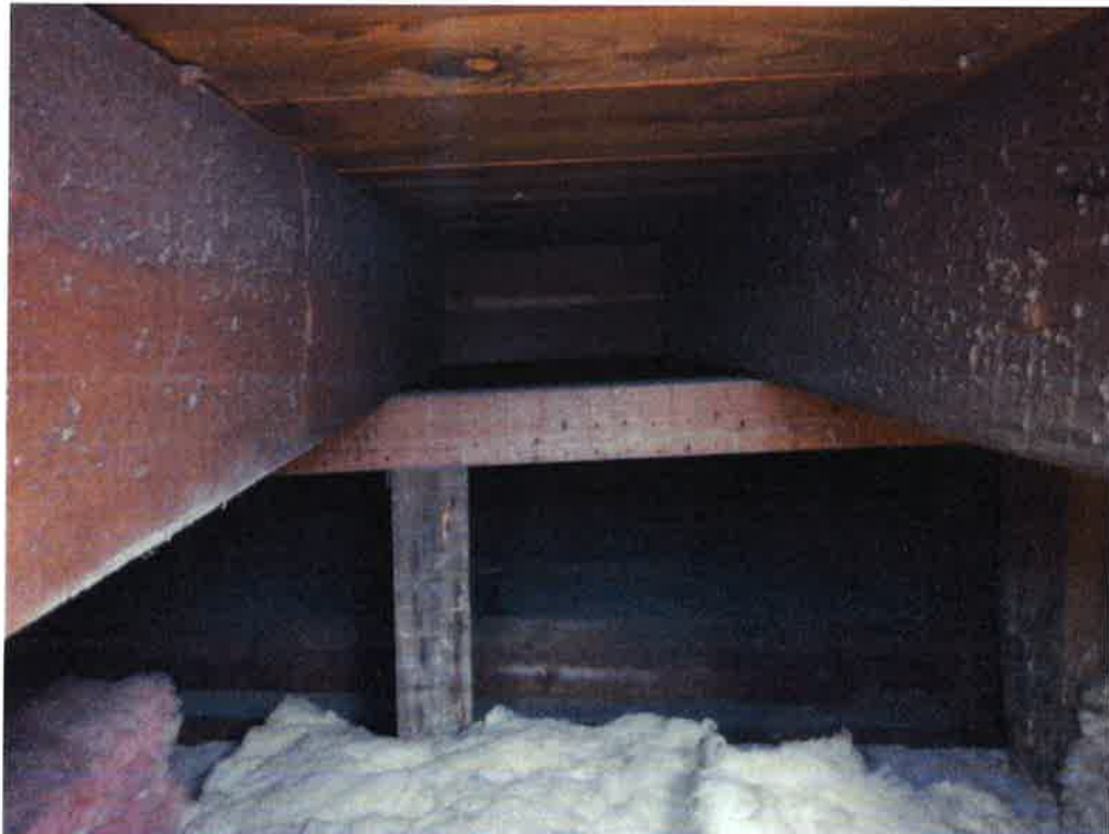
Photo 2: Sample photo showing the existing roof construction below the FRP chimney.
