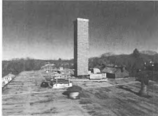
Photo 1: Sample photo showing the existing ballasted chimney.
