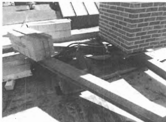
Photo 2: Sample photo showing the existing ballasted frame.
