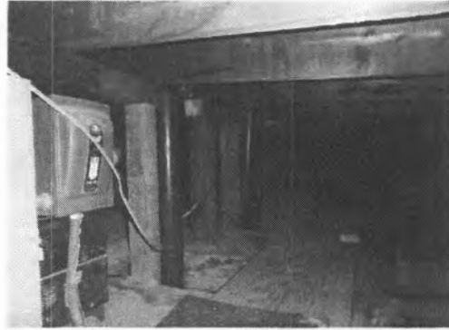
Photo 6: Sample photo showing the existing roof structure.
