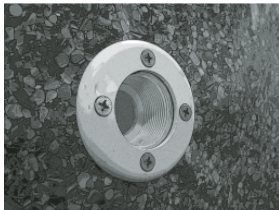
Return faceplate installed.
