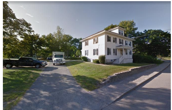
Figure 3: Single-family structure to be demolished under proposed expansion.
