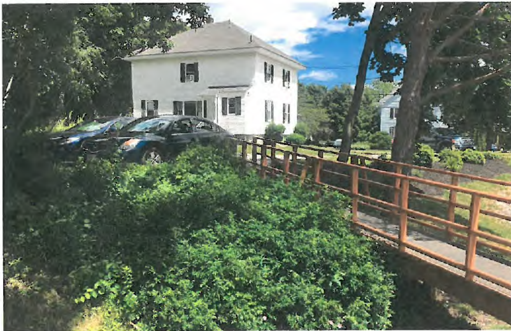
Looking to the Northeast from the entrance drive. The building will overlap the rear portion of the white building.
