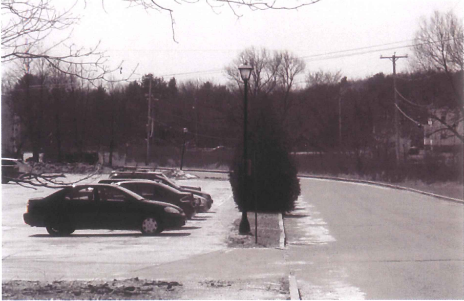
Photo 5: Pheasant Hill Rd. – no sidewalk along parking lot
