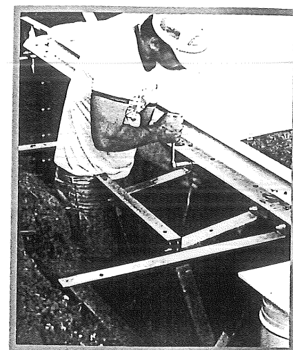
8. Ladder supports are fastened.
