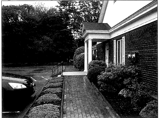
Figure 2: Existing Structure Side Entrance
