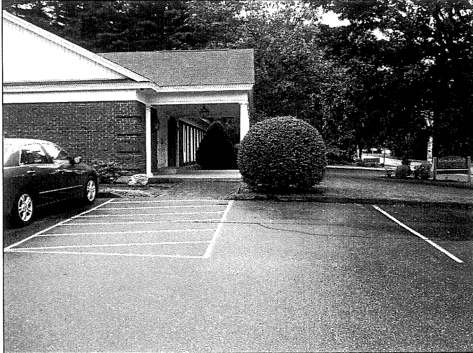
Figure 1: Existing Structure Lobby Entrance
