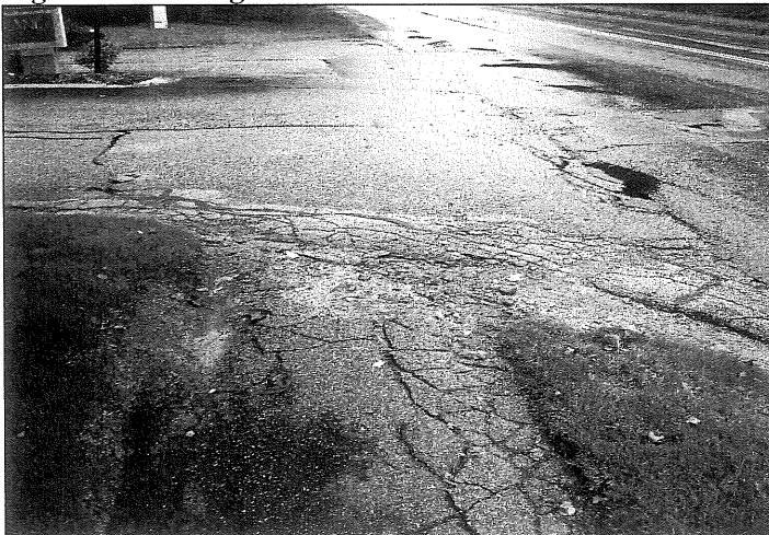
Figure 5: Existing sidewalk condition at Tamarlane
