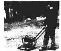
Using a plate compactor to pack the gravel
