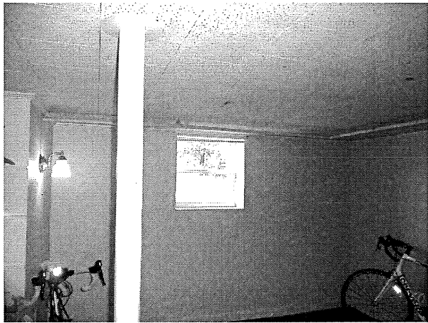
Photo #4 – Basement window near north end of west endwall
