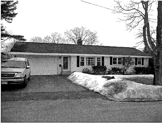
Photo # 1 – North elevation
