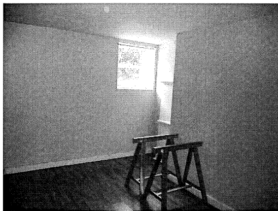
Photo # 5 – Basement window at middle of west endwall
