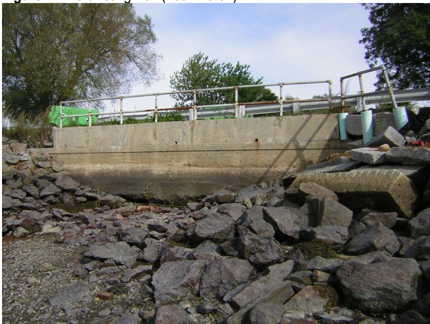
Figure 2. The existing wall (2007-10-02)
