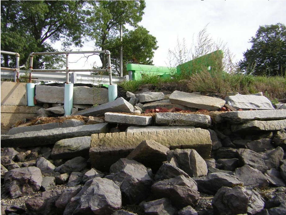
Figure 3. Riprap and granite blocks adjacent to retaining wall (2007-10-02)
