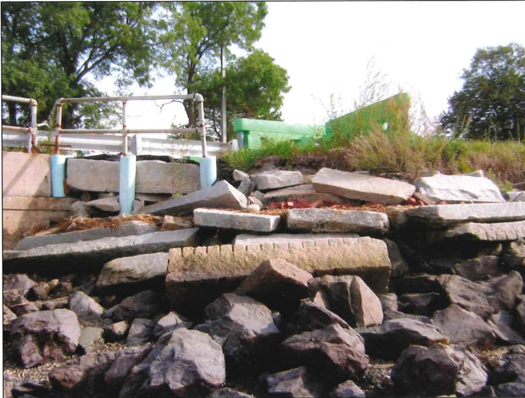
Photo 3: Riprap and granite blocks adjacent to retaining wall (2007-10-02).
