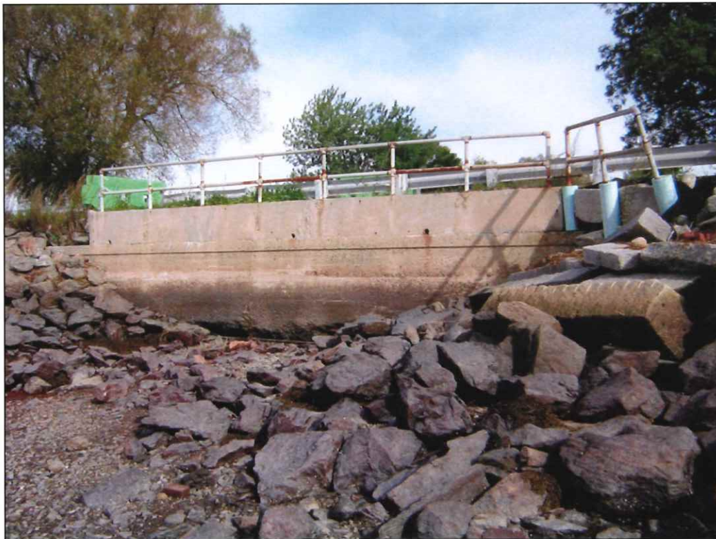
Photo 2: The existing wall (2007-10-02).
