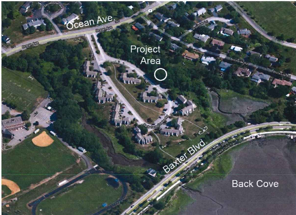
Back Cove Estates is located just above Back Cove. The development is located between Ocean Ave, Baxter Blvd & two streams. The project area is shown on the above aerial photo.
