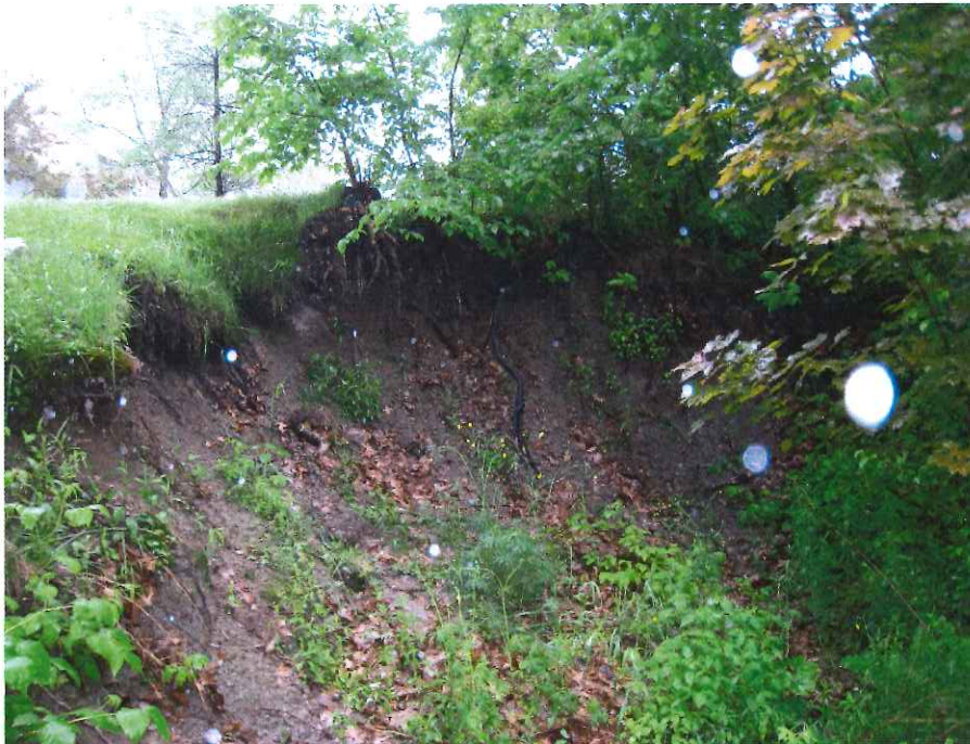
A 6'-8' high vertical face is located along the upper rim of the slide.
