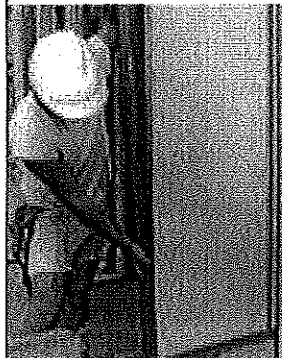
USG STEEL H-stud slides in place over SHEETROCK Brand Gypsum Liner Panels.
