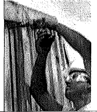
USG Aluminum Breakaway Clip is screw-attached to studs and framing. Under fire exposure, clip breaks away, permits fire-damaged wall to fall, leaving separation wall intact.
