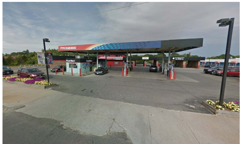
Figure 2: View of the site through the central curb cut. Note, the 'food mart' structure and portion of the canopy directly overhead is to be removed.
