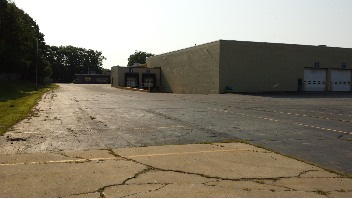
Photo 1: Existing Site Conditions
