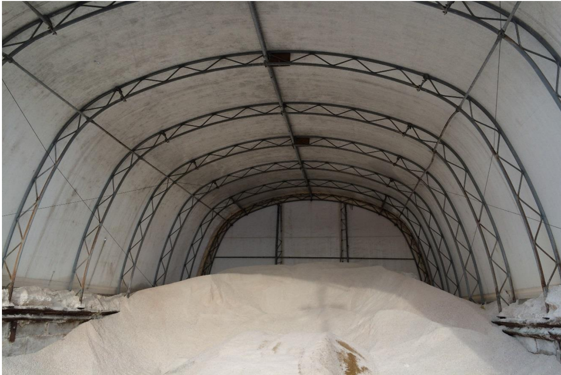
Photo 2: Inside of existing salt shed located on Hanover Street in Portland.
