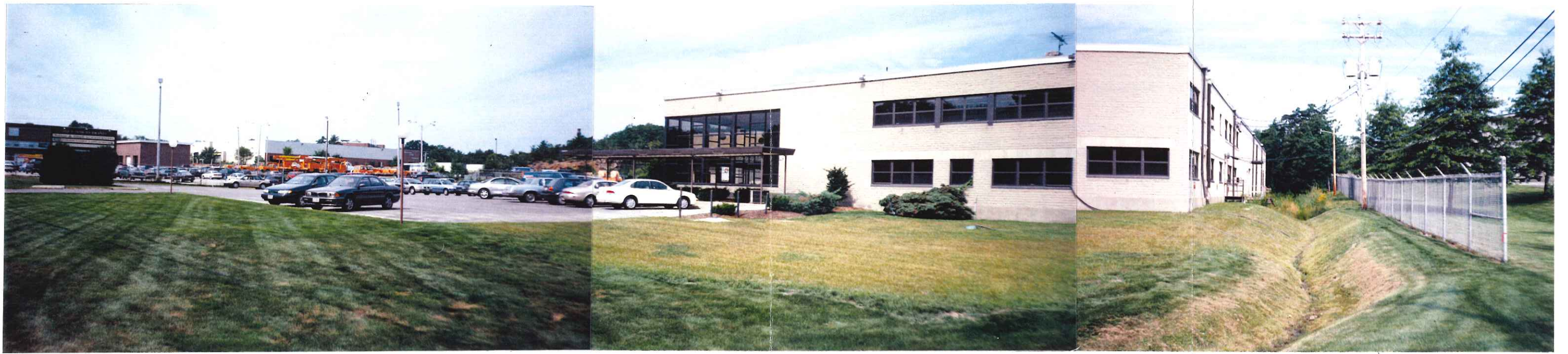
VIEW FROM EASTERN CORNER OF SITE
