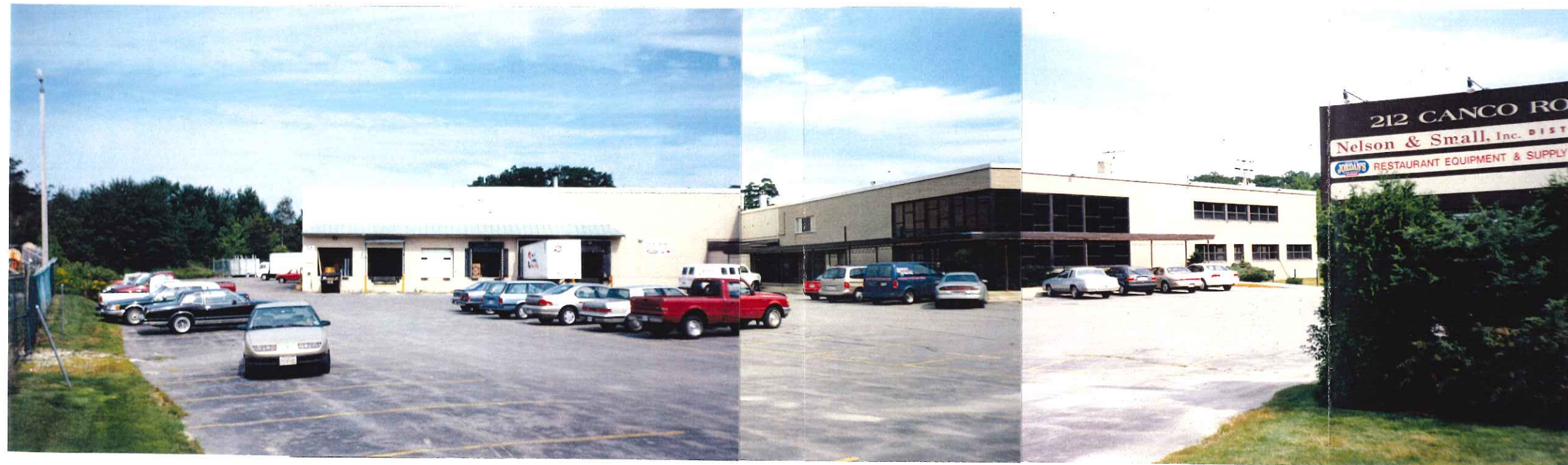
VIEW FROM SOUTHERN CORNER OF SITE
