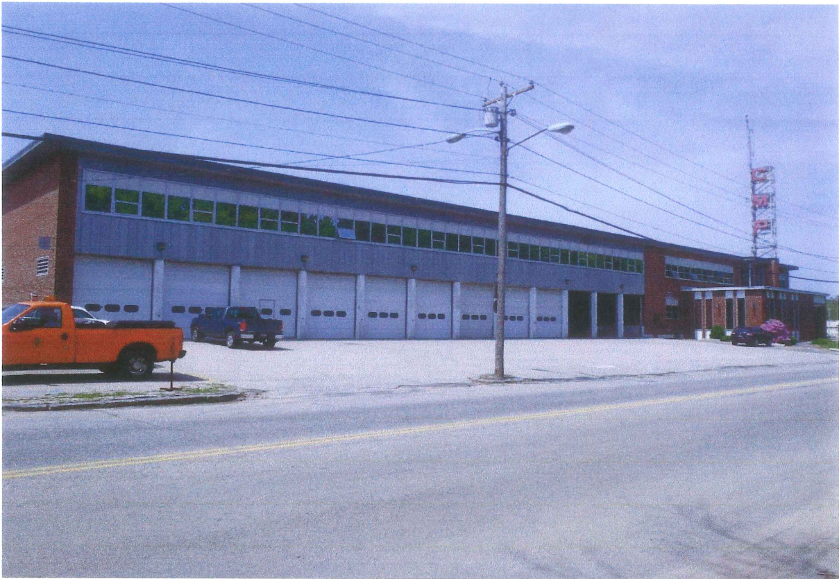
138 Canco Road Portland. Existing East Truck with 12 overhead doors facing Canco Road. New addition will be out 5'-6" toward Canco Road to provide storage space for new longer line trucks.
