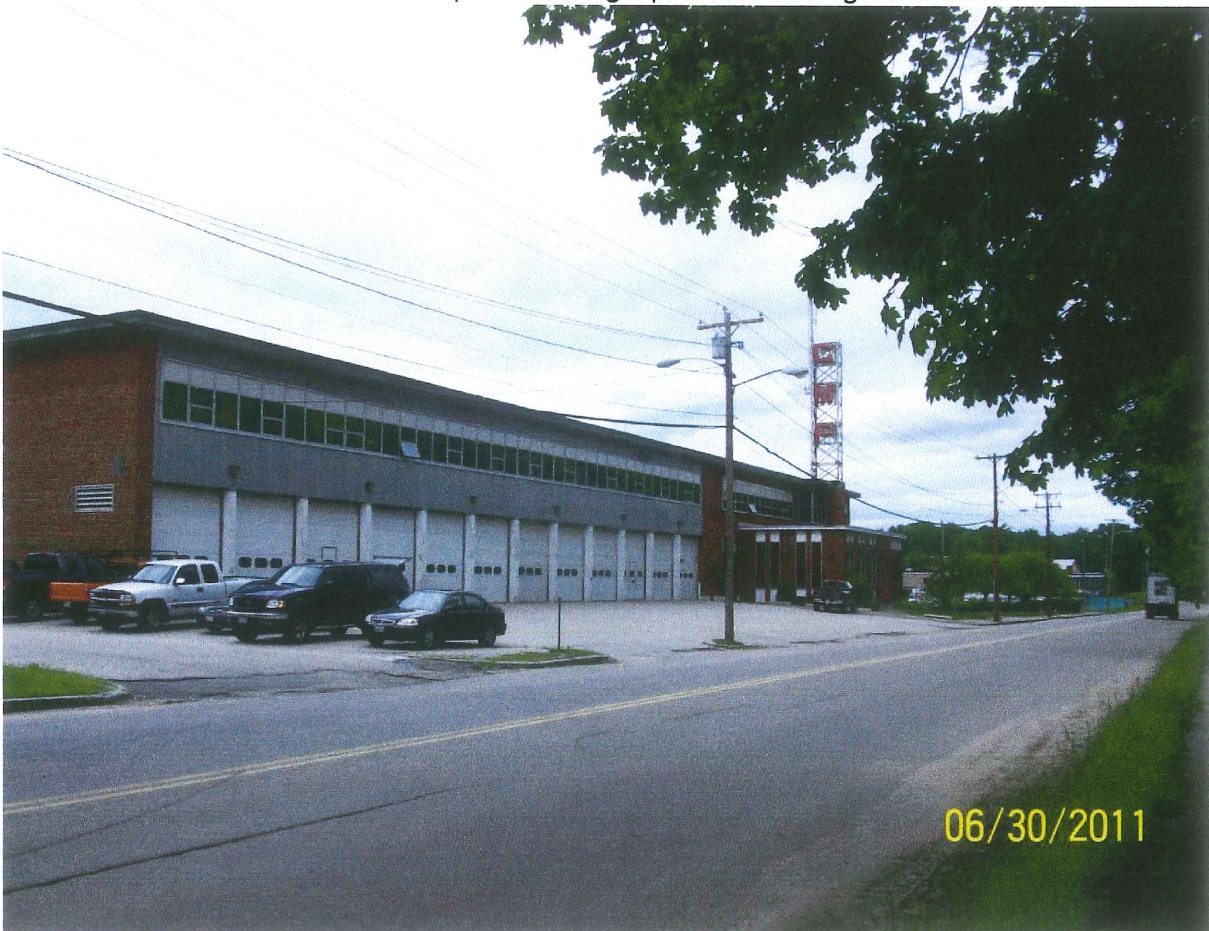
138 Canco Road Portland. Existing East Truck with 12 overhead doors facing Canco Road. New addition will be out 5'-6" toward Canco Road to provide storage space for new longer line trucks.
