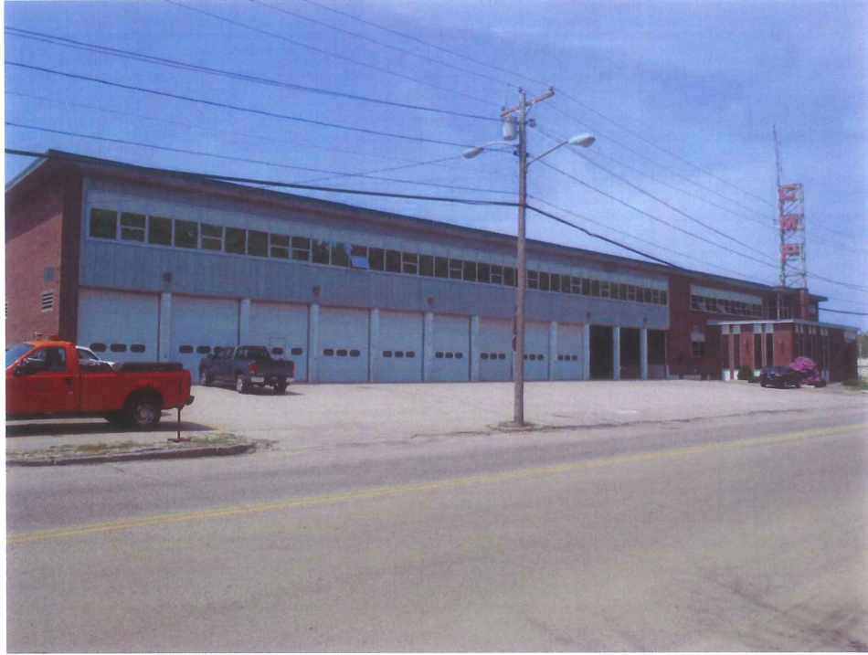
06-08-11 138 Canco Road Portland. Existing East Truck with 12 overhead doors facing Canco Road. New addition will be out 5'-6" toward Canco Road to provide storage space for new longer line trucks.
