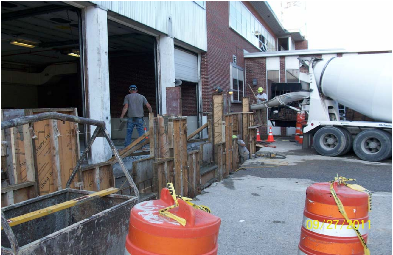
09-27-11 Placing concrete at new addition north wall.
