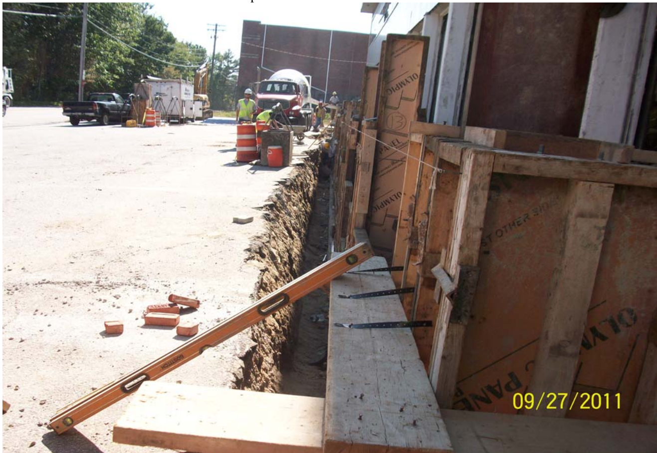
09-27-11 Placing concrete at new addition south wall.
