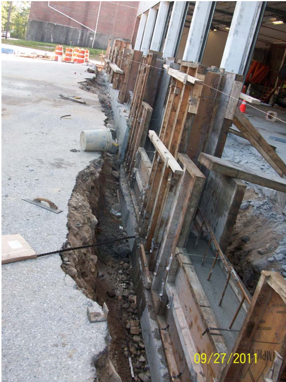
09-27-11 Concrete in place.
