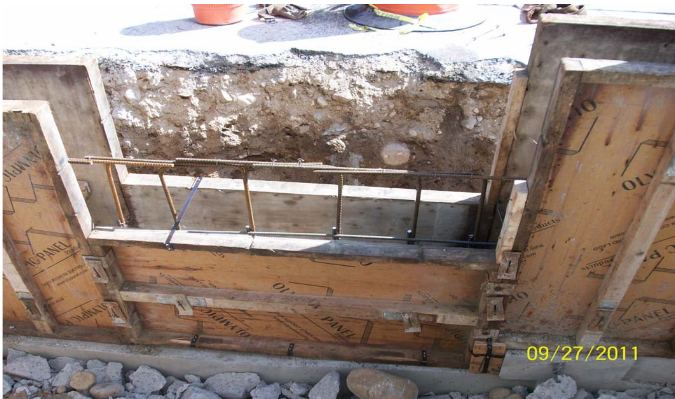
09-27-11 Formwork and recess in wall to accept new slab.
