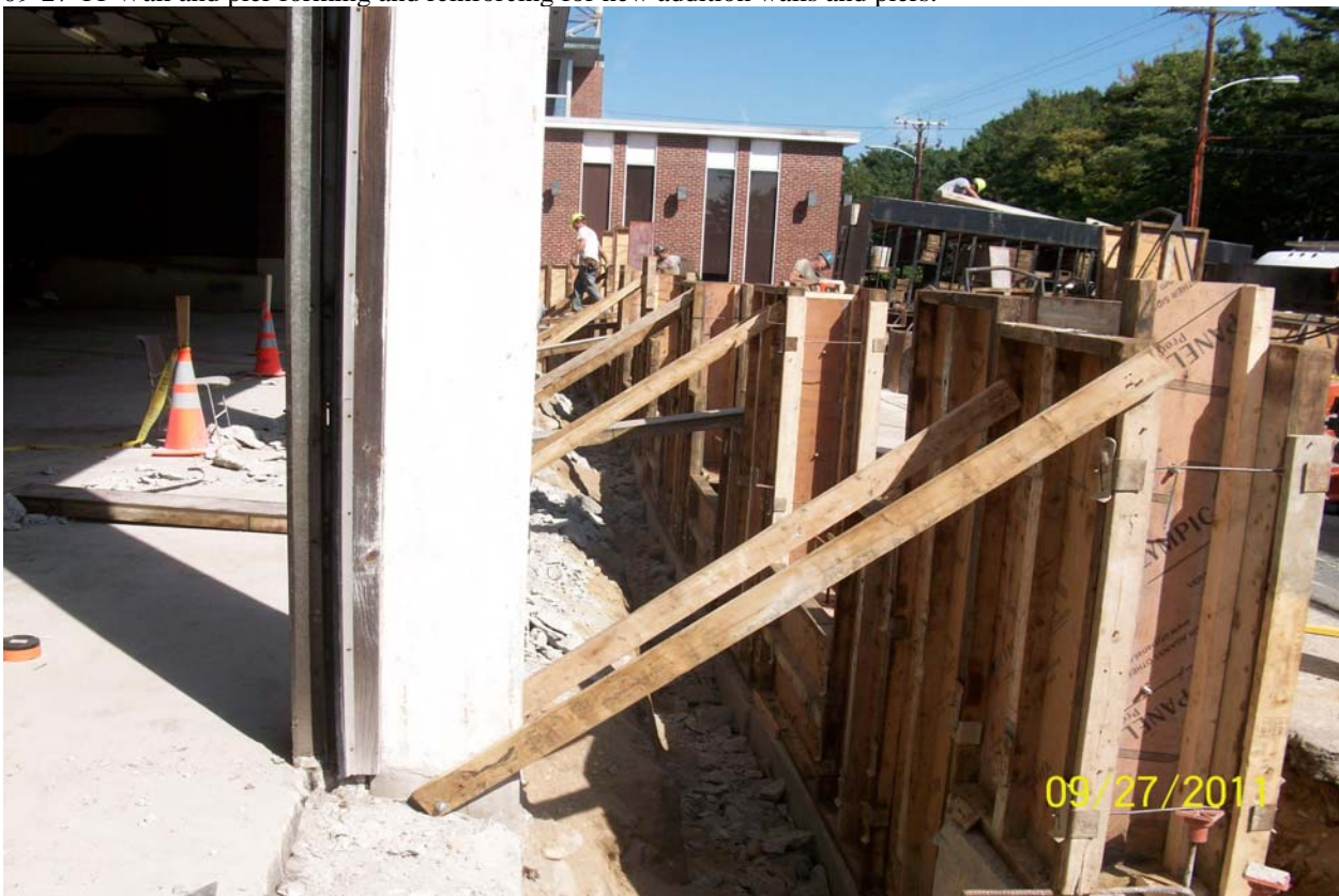
09-27-11 Bracing of pier forms.
