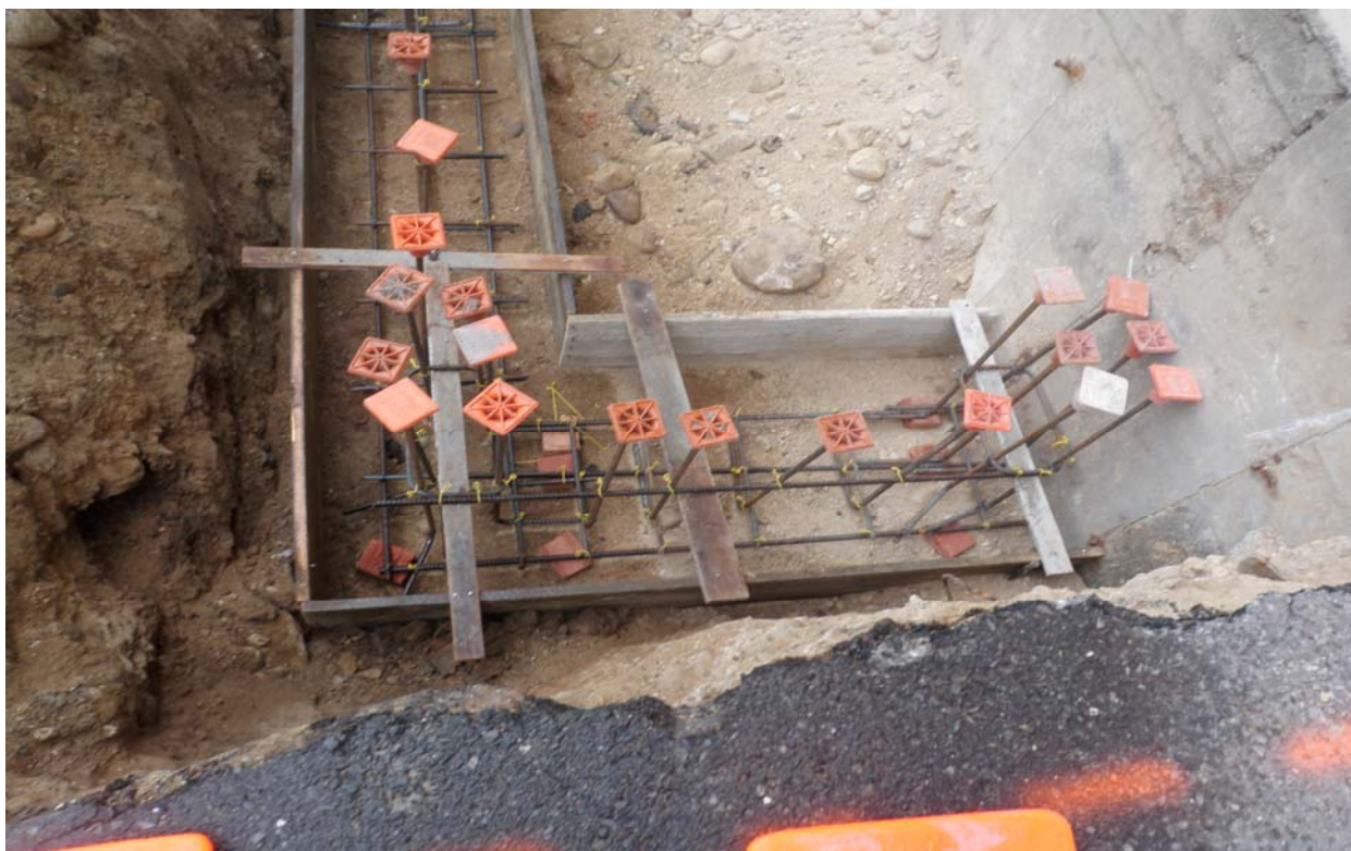
09-20-11 Forming and reinforcing for new addition footing.
