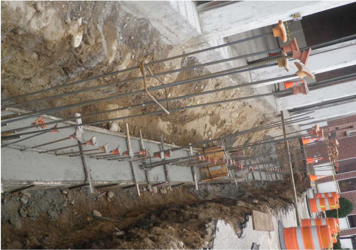
09-23-11 Concrete footing placed.
