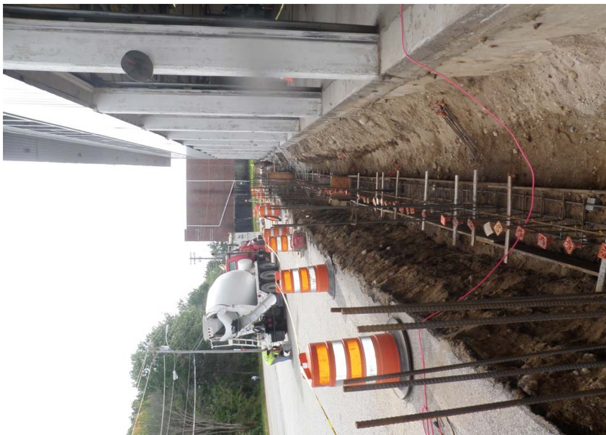
09-23-11 Forms and reinforcing in-place ready for concrete placement.
