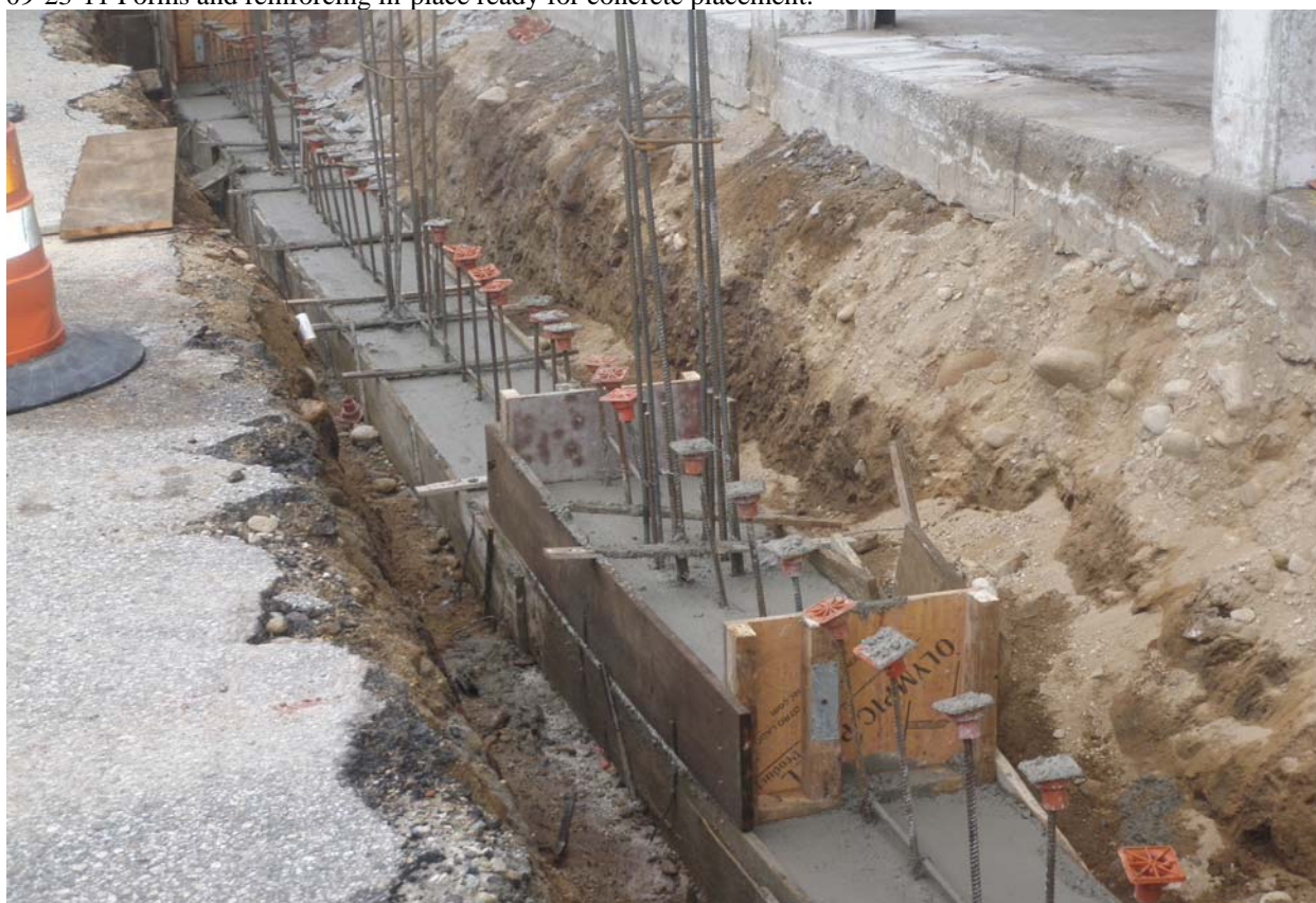
09-23-11 Concrete footing placed.
