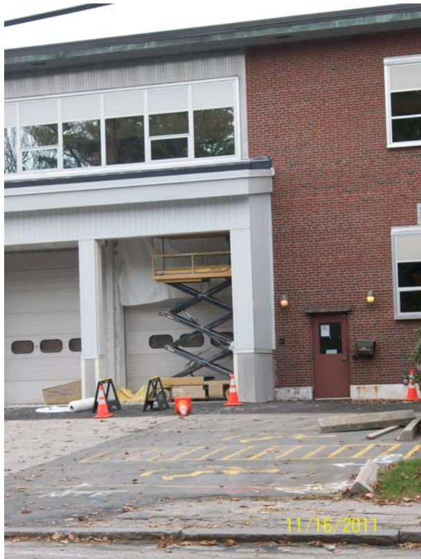
11-16-11 north end wall exterior view.
