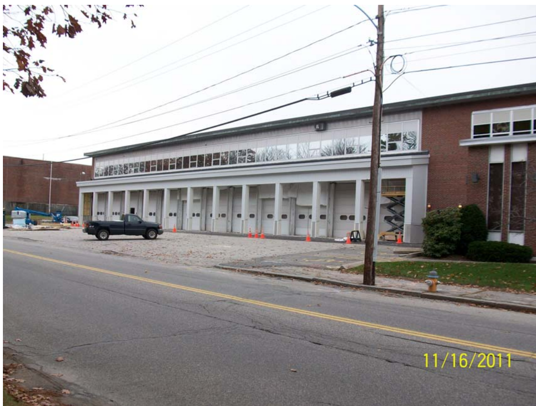
11-16-11 overview of entire site
