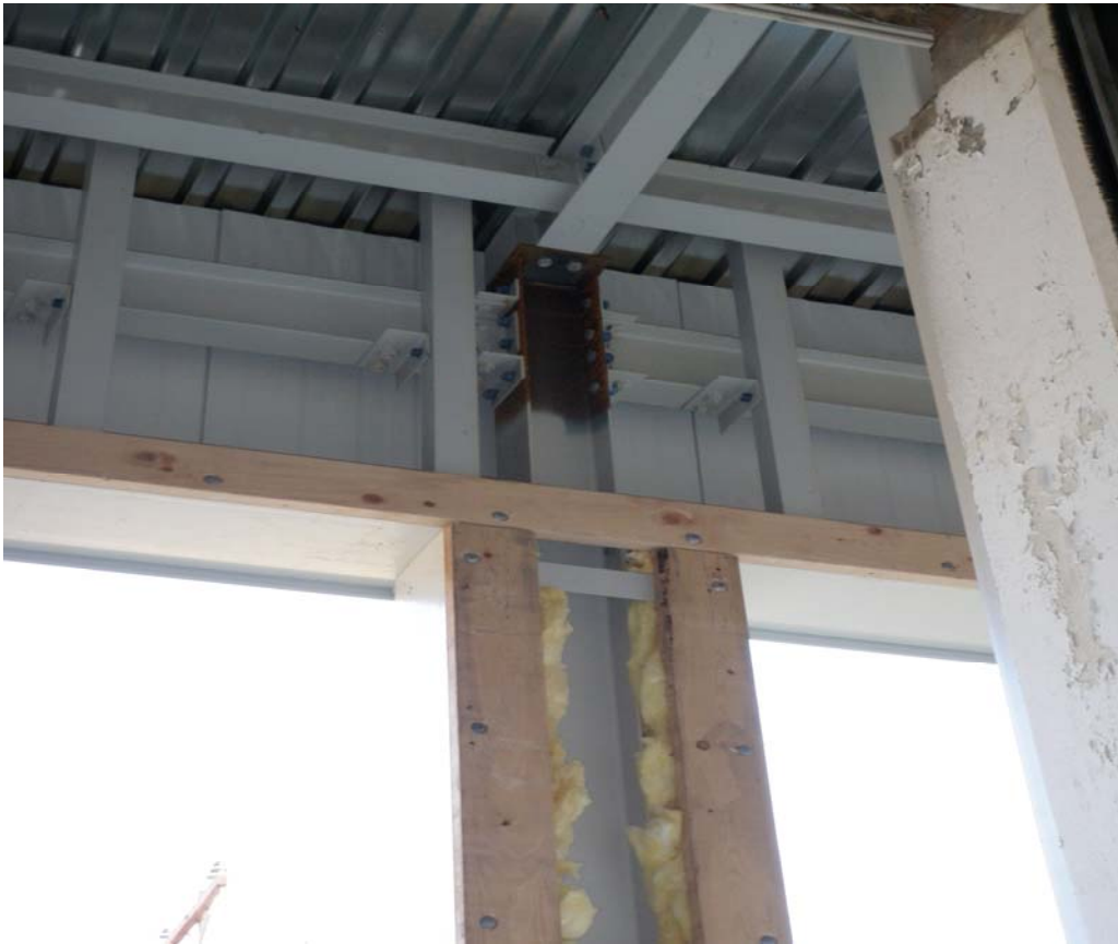
11-09-11 door bucks and insulation installed between overhead doors, plywood is cut and waiting to be painted.
