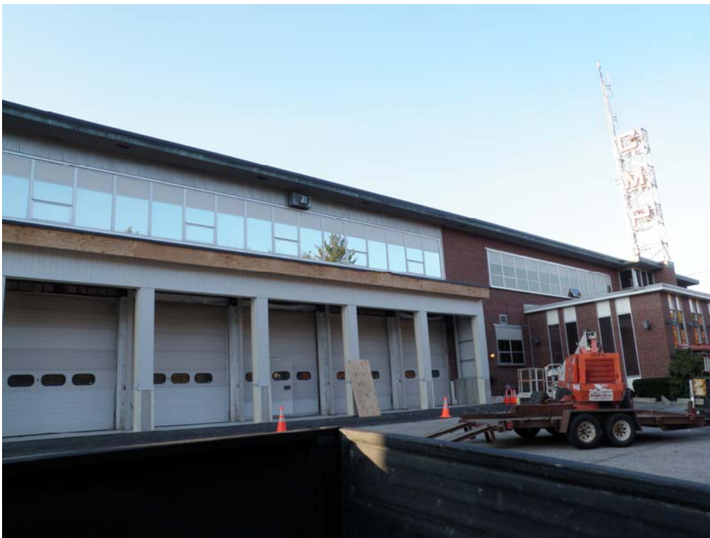
11-09-11 all of the siding is on and the roof membrane is glued down no aluminum fascia on this section.
