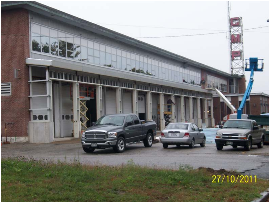
10-28-11 all of steel is up and roof decking is in place
