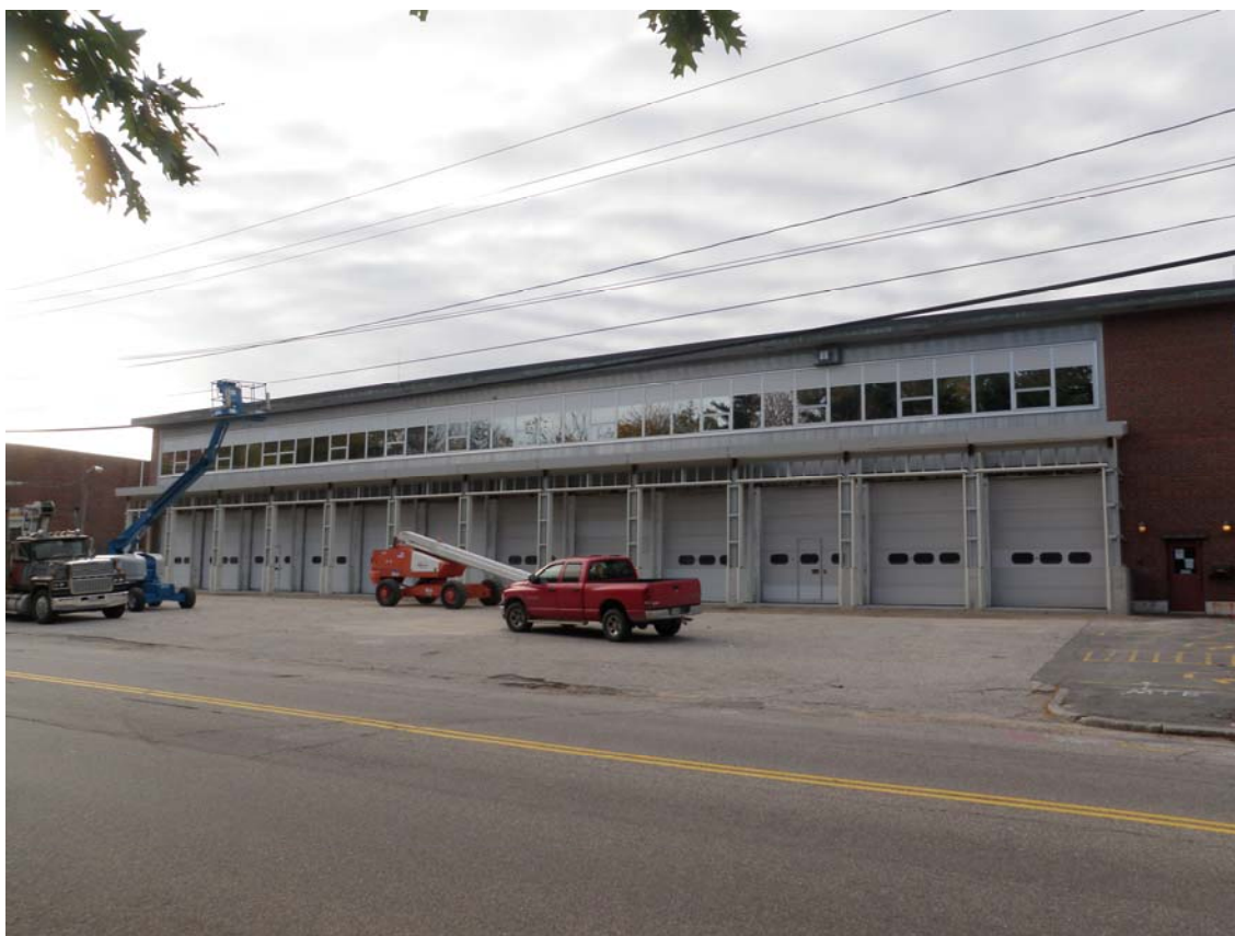
10-26-11 overview of entire site
