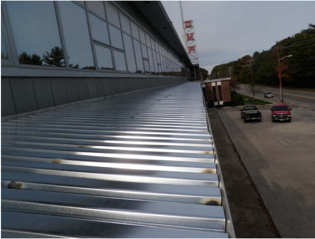
10-26-11 Steel roof deck in place
