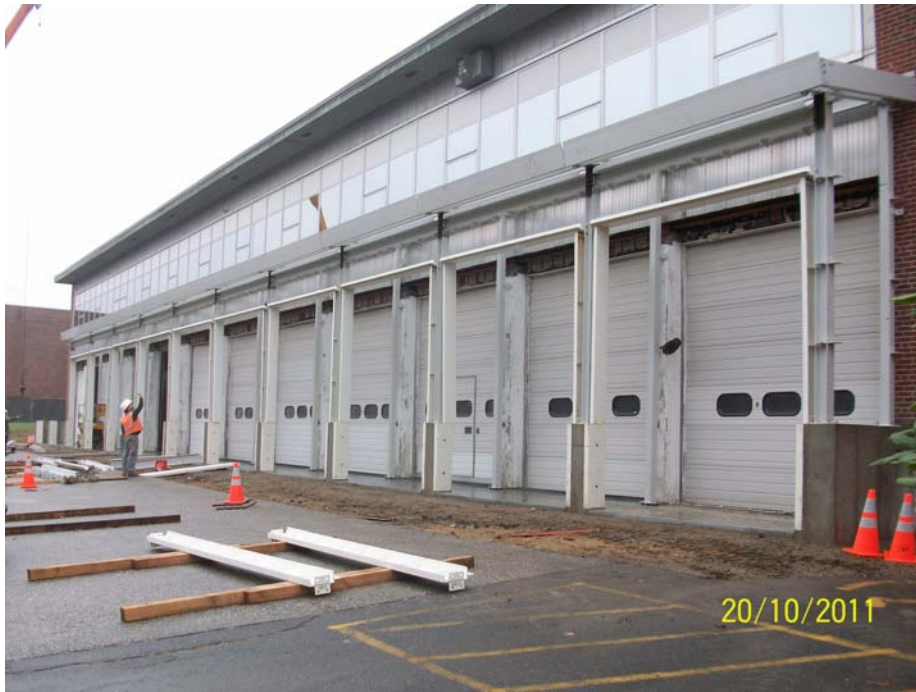
10-20-11 overview of the new addition 10 out of 12 bays erected.
