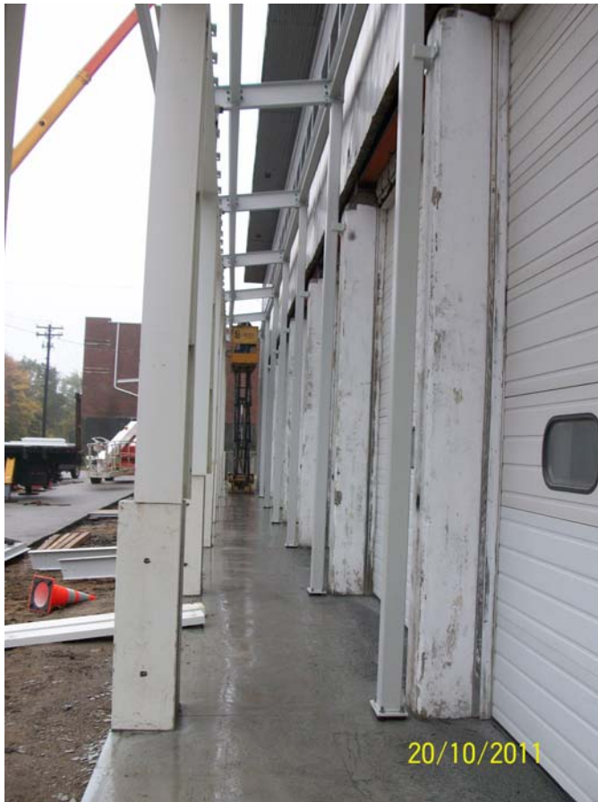
10-20-11 saw looking down the new addition.
