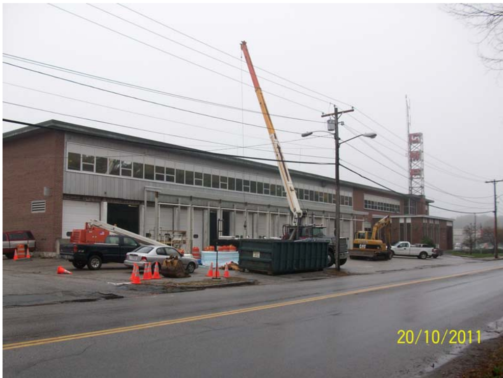
10-20-11 overview of entire site during steel erection.
