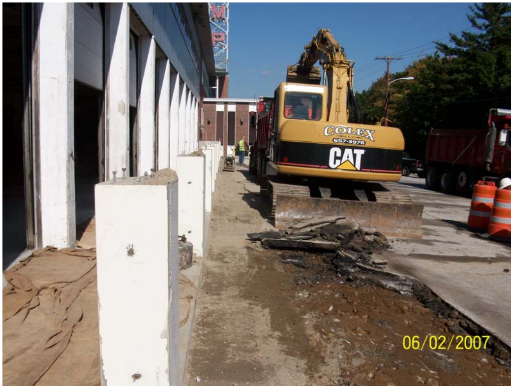
10-10-11 saw cutting and removing the existing pavement.
