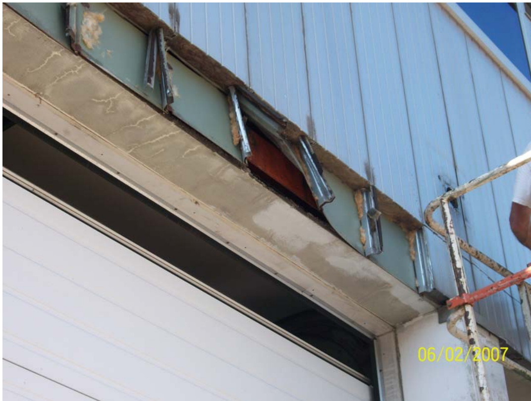
10-10-11 siding being removed.
