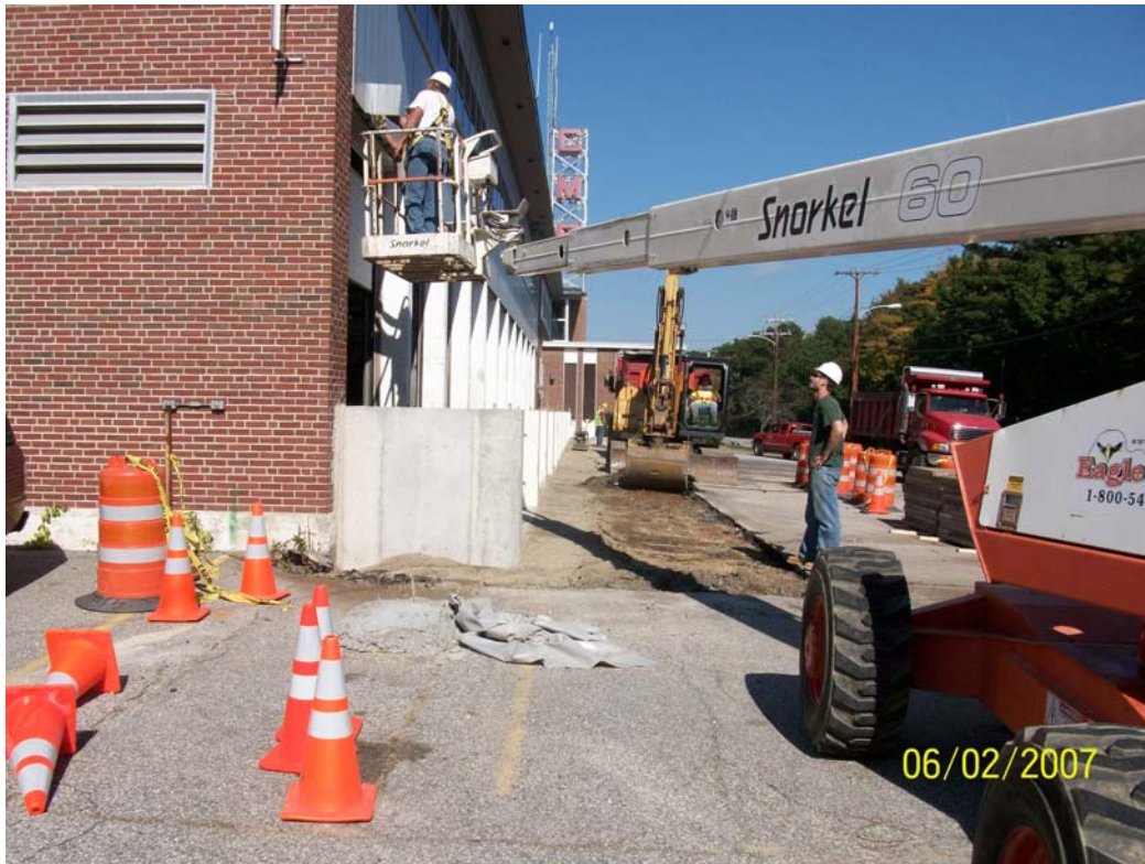
10-10-11 working on saw cutting and removing the required section of siding.
