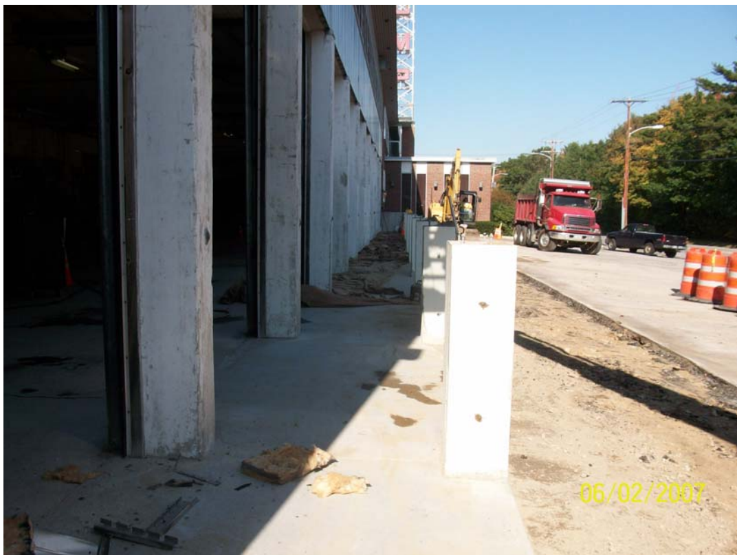
10-10-11 slab complete still covered with burlap from wet curing.
