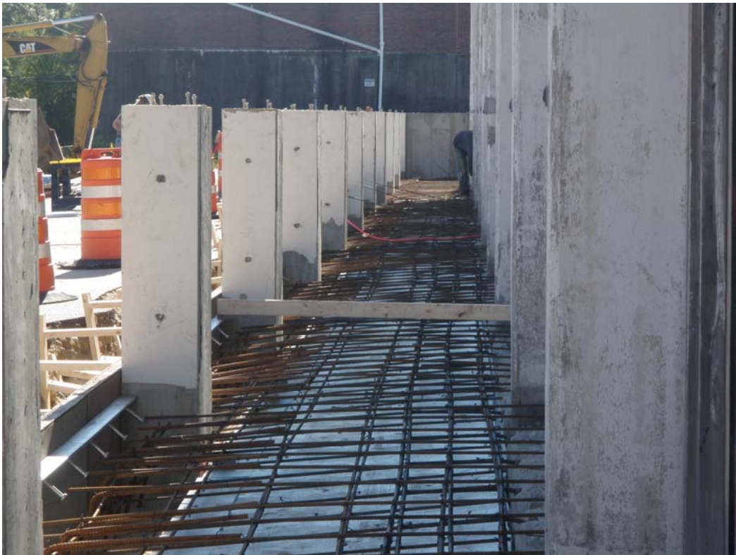
10-06-11 slab forming and reinforcing for new addition slab.
