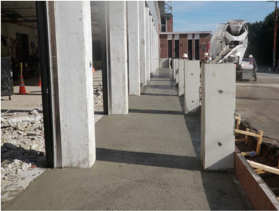
10-07-11 placing concrete for addition slab.
