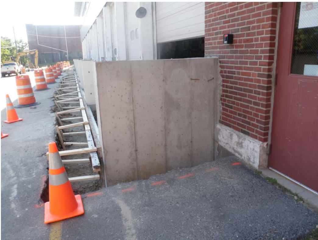
10-06-11 bracing of slab forms.
