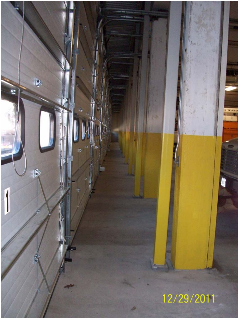
12-29-11 looking down the interior of the new addition.
