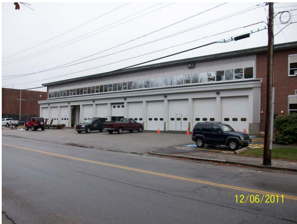
12-06-11 overall view of the new addition from the right.
