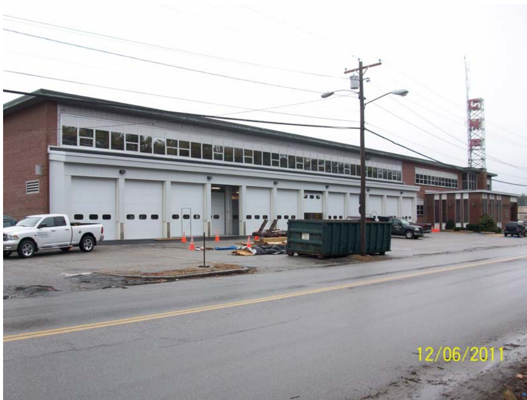
12-06-11 overall view of the new addition from the left.
