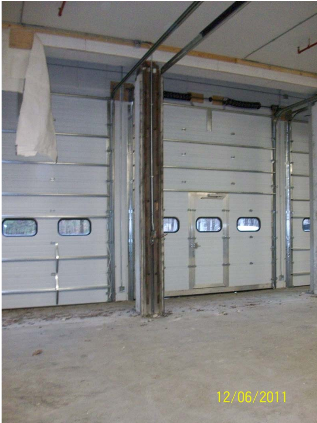
12-06-11 Interior view of new overhead doors stacked & existing doors removed.
