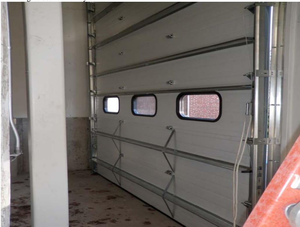
12-02-11 interior new overhead doors assembled & stacked.
