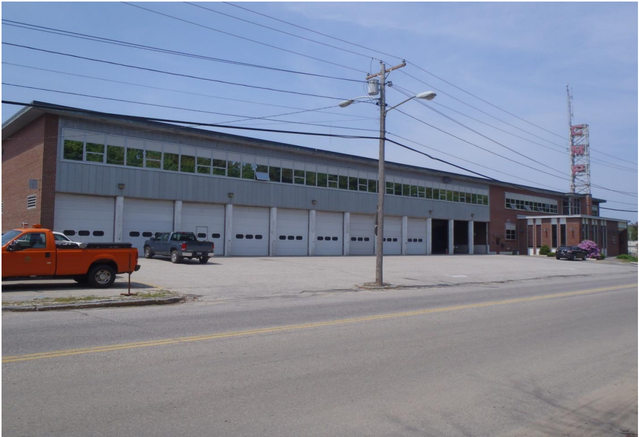
138 Canco Road Portland. Existing East Truck with 12 overhead doors facing Canco Road. New addition will be out 5'-6" toward Canco Road to provide storage space for new longer line trucks.
