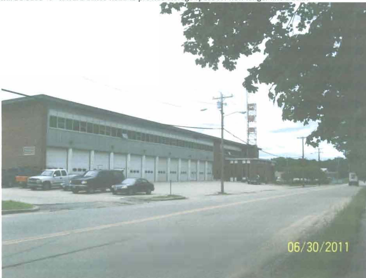
138 Canco Road Portland. Existing East Truck with 12 overhead doors facing Canco Road. New addition will be out 5'-6" toward Canco Road to provide storage space for new longer line trucks.
