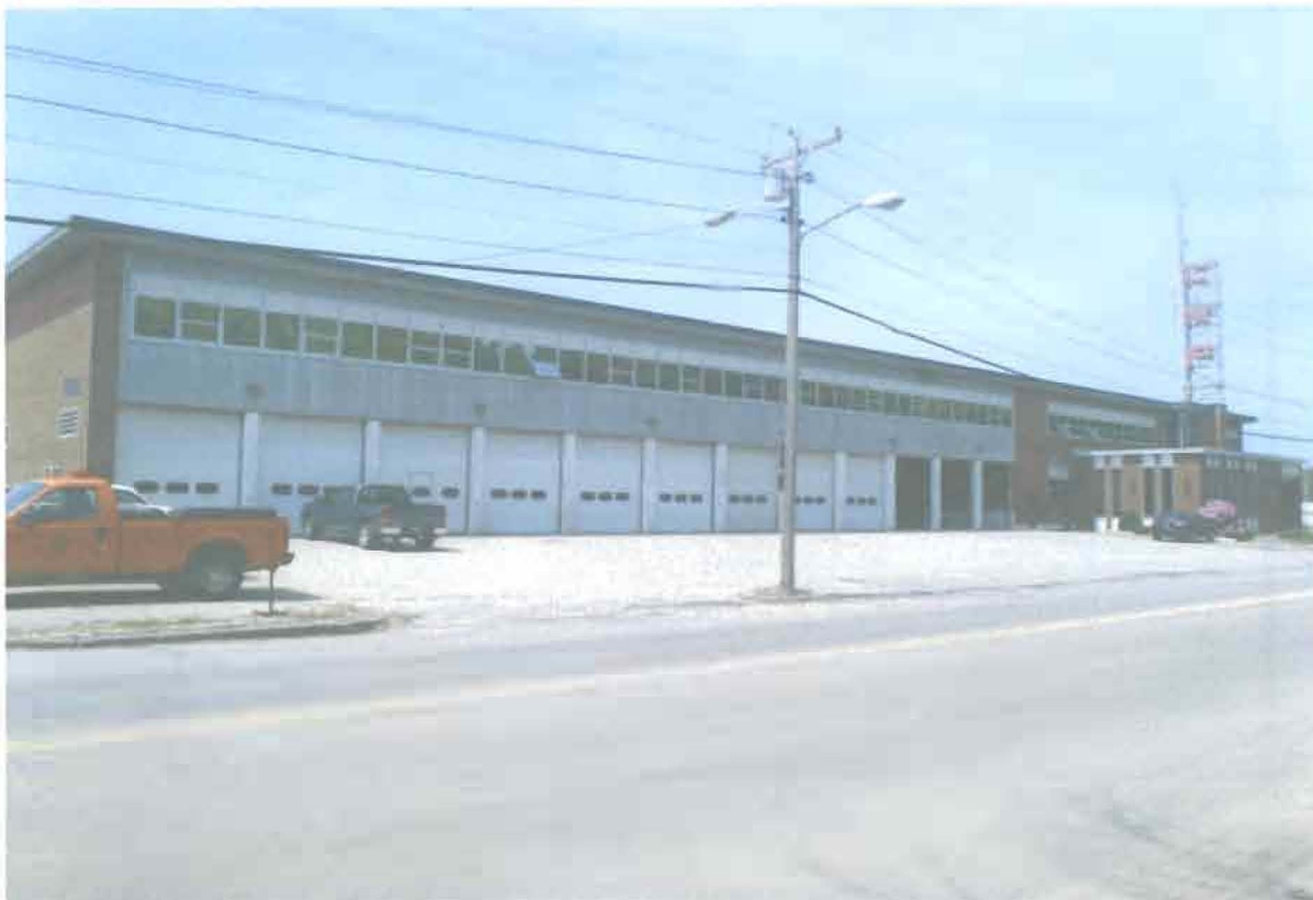
138 Canco Road Portland. Existing East Truck with 12 overhead doors facing Canco Road. New addition will be out 5'-6" toward Canco Road to provide storage space for new longer line trucks.
