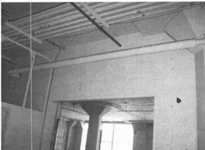
Hard-pack insulation observed overhead on first floor (sample 14A)
