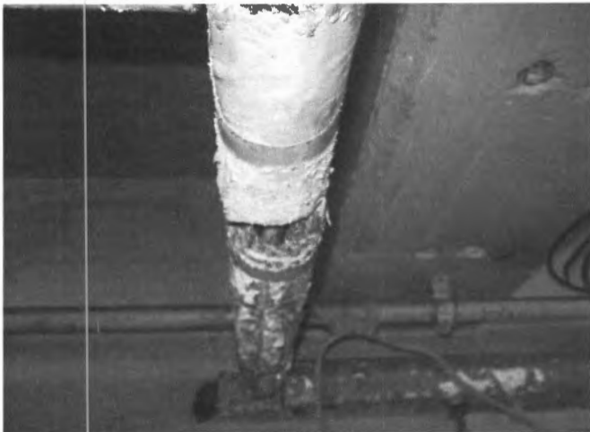
Corrugated pipe insulation observed in basement (sample 02A)
