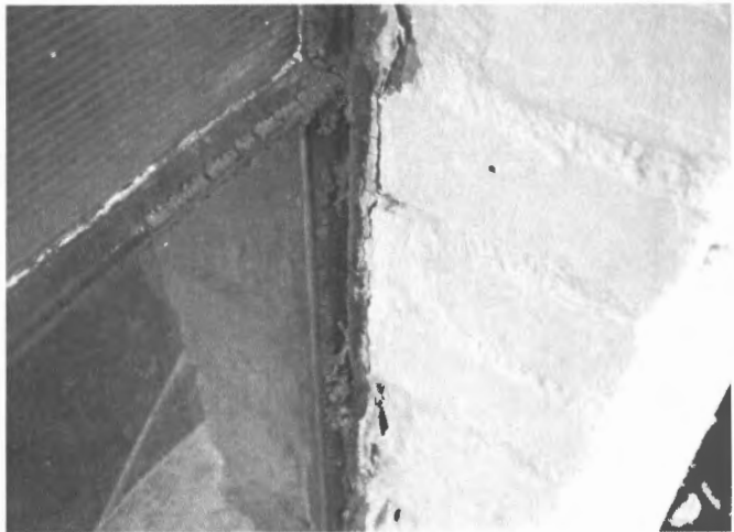
Exterior window caulk (sample 18A)
