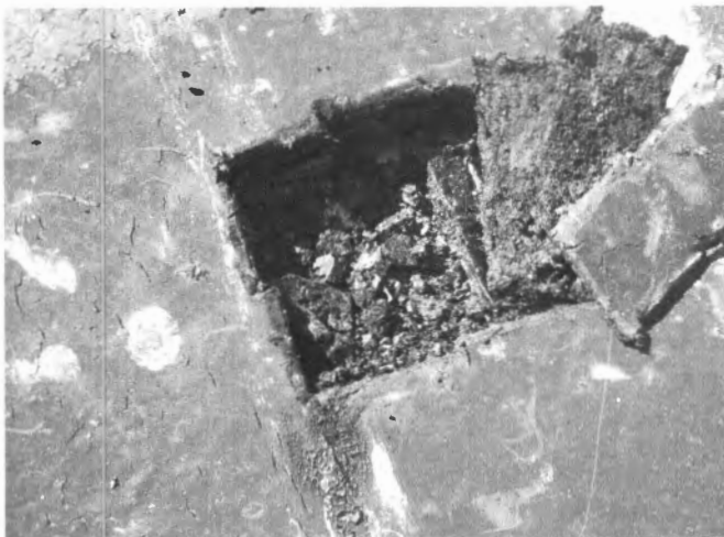
Closer view of vaulted roof section core cut (sample R-02A)
