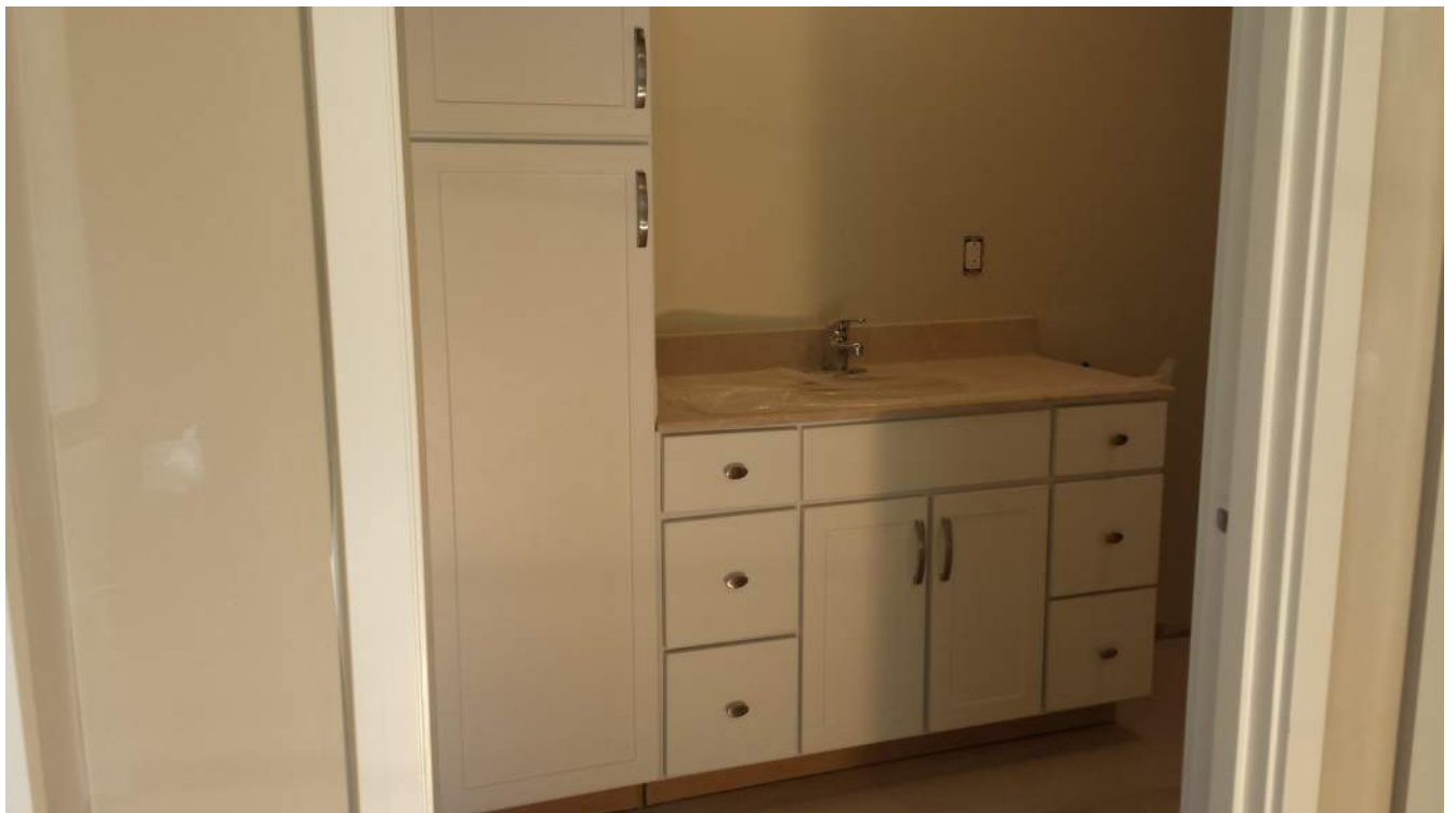
Levels 3 & 4 Typical Unit progress (Unit 1401 shown).
