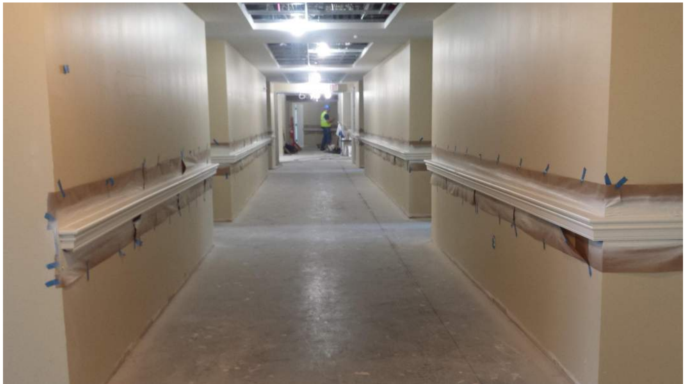
Level 2 New Construction East Wing
