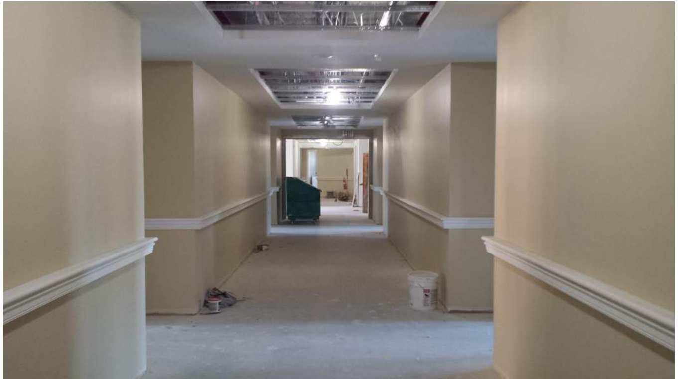
Level 3 New Construction West Wing
