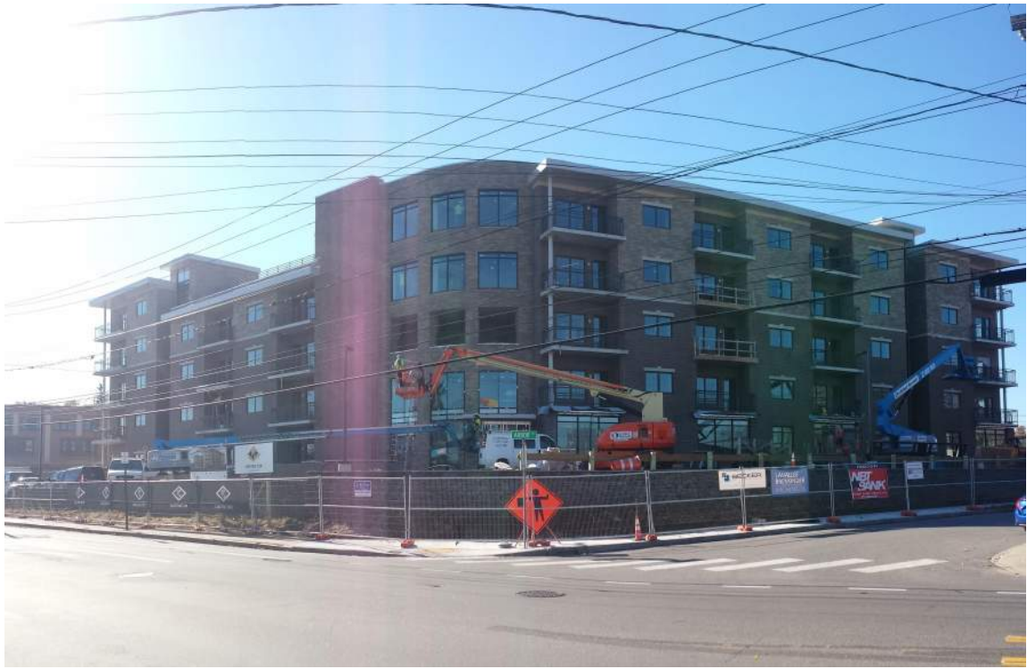
New Construction at Forest Ave and Arbor Street
