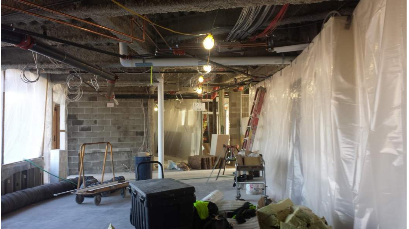
Connector typical progress (corridor 141 shown)
