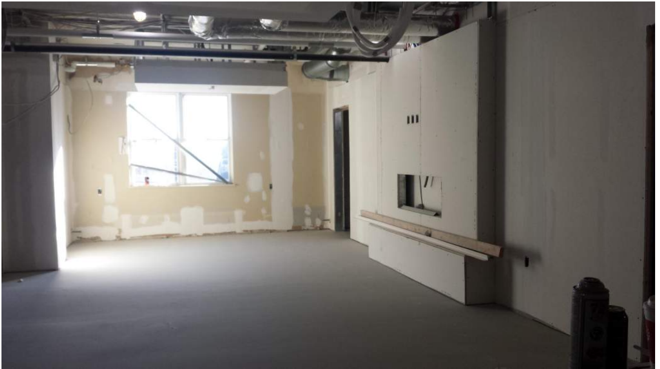
Main Street typical room progress (Pub 125 shown)
