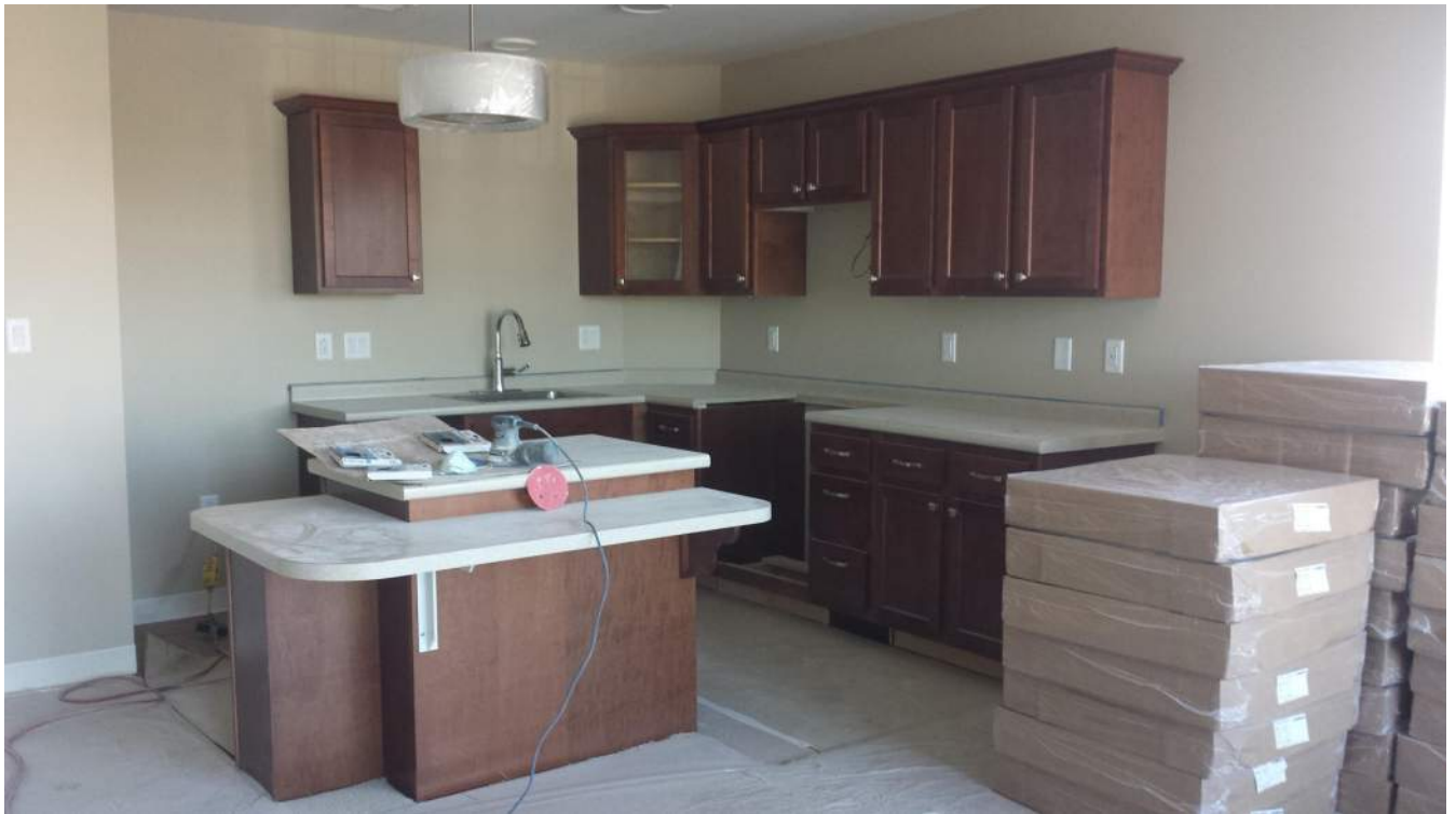
Levels 3 & 4 Typical Unit progress (Unit 1300 shown).
