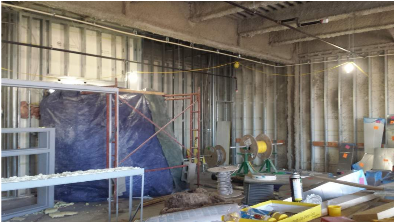
Connector typical room progress (Auditorium 132 shown)
