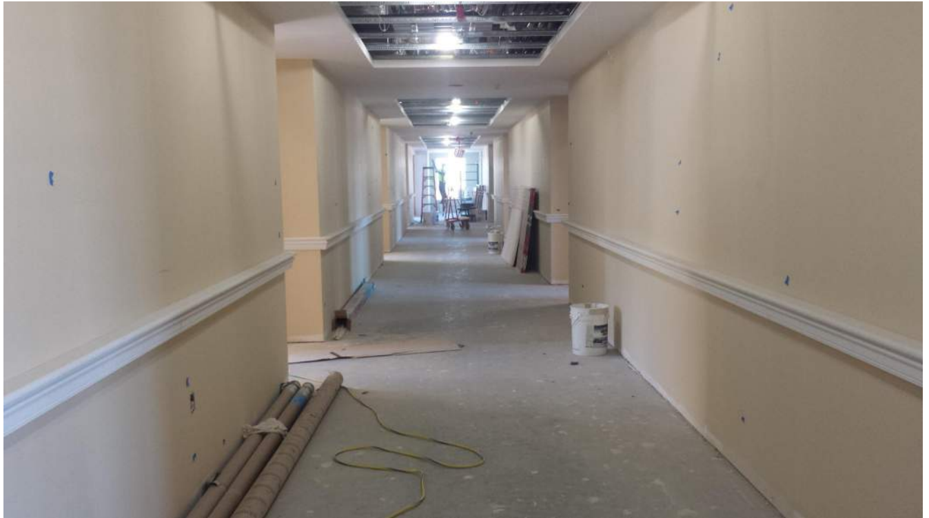
Level 4 New Construction West Wing
