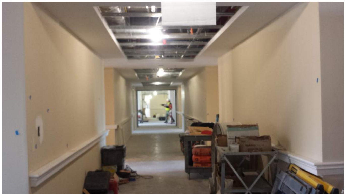
Level 4 New Construction East Wing
