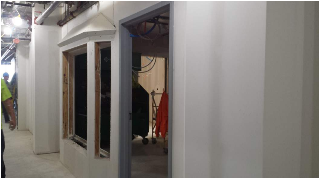
Main Street typical corridor progress
