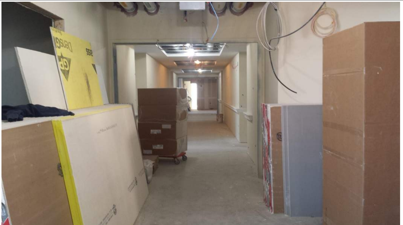
Level 1 New Construction East Wing
