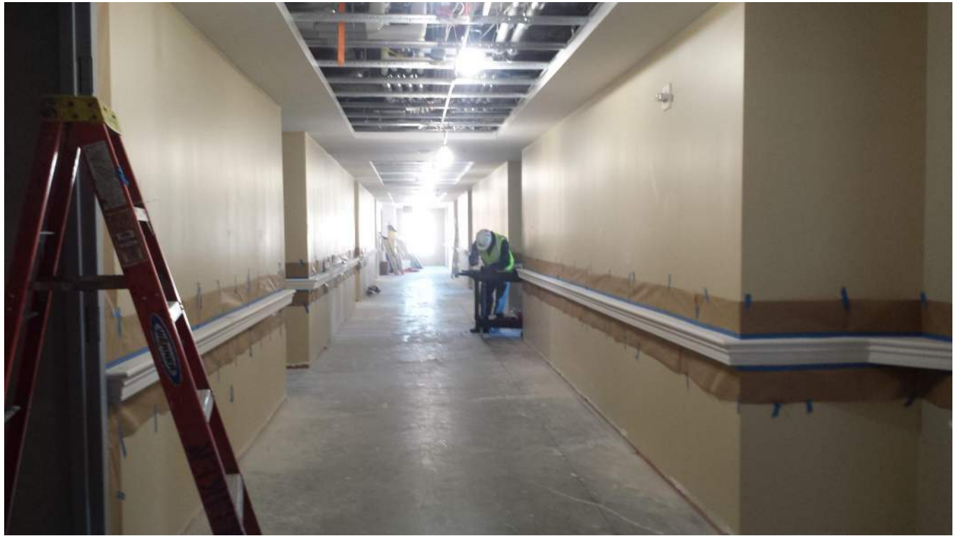
Level 2 New Construction West Wing
