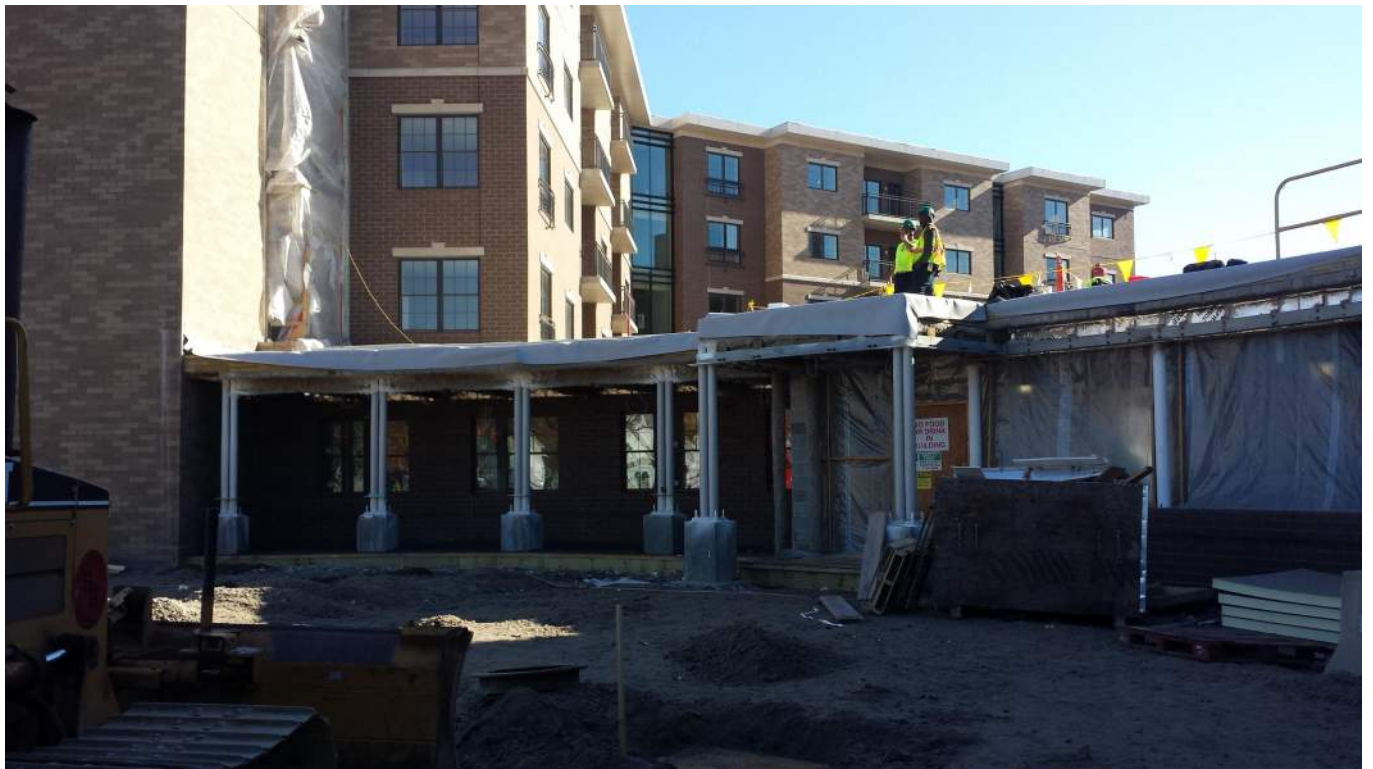
Renovation Main Street Courtyard Side
