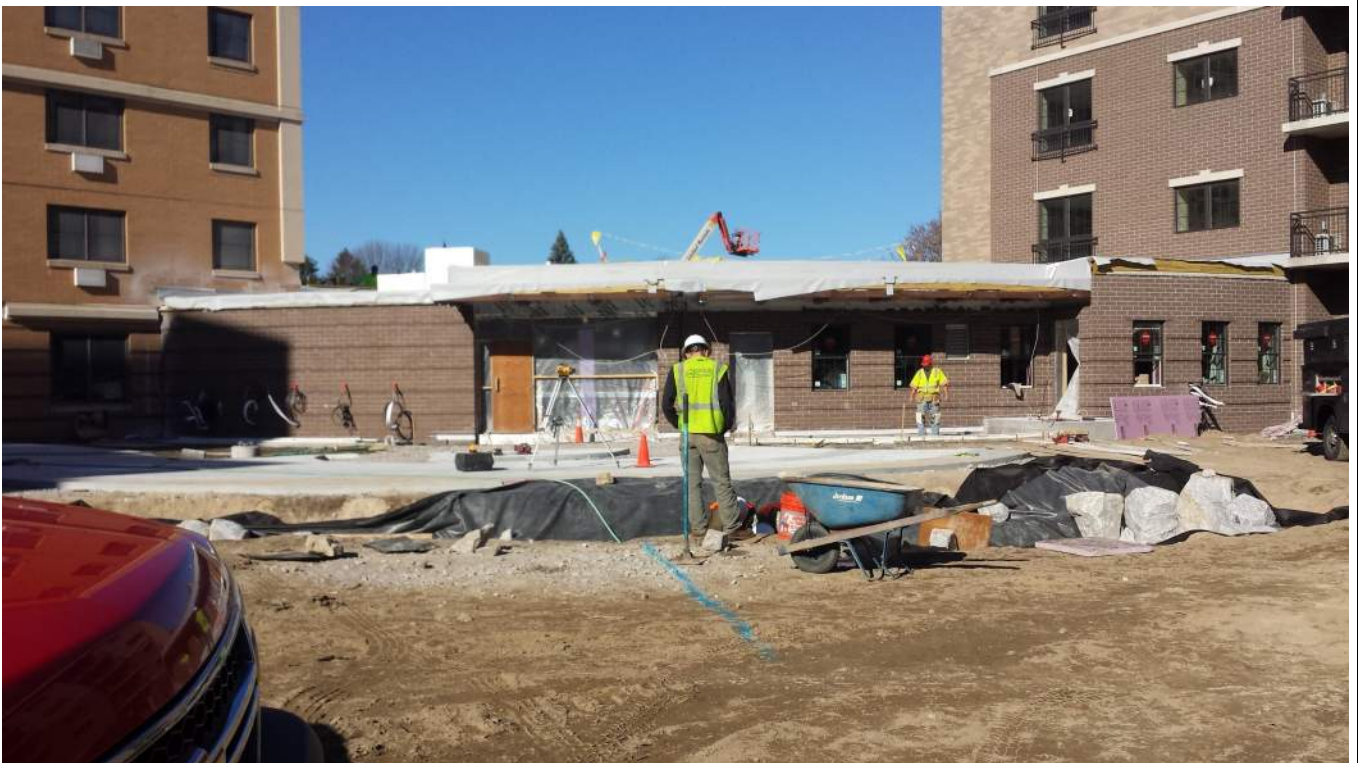
New Construction Connector, Courtyard Side
