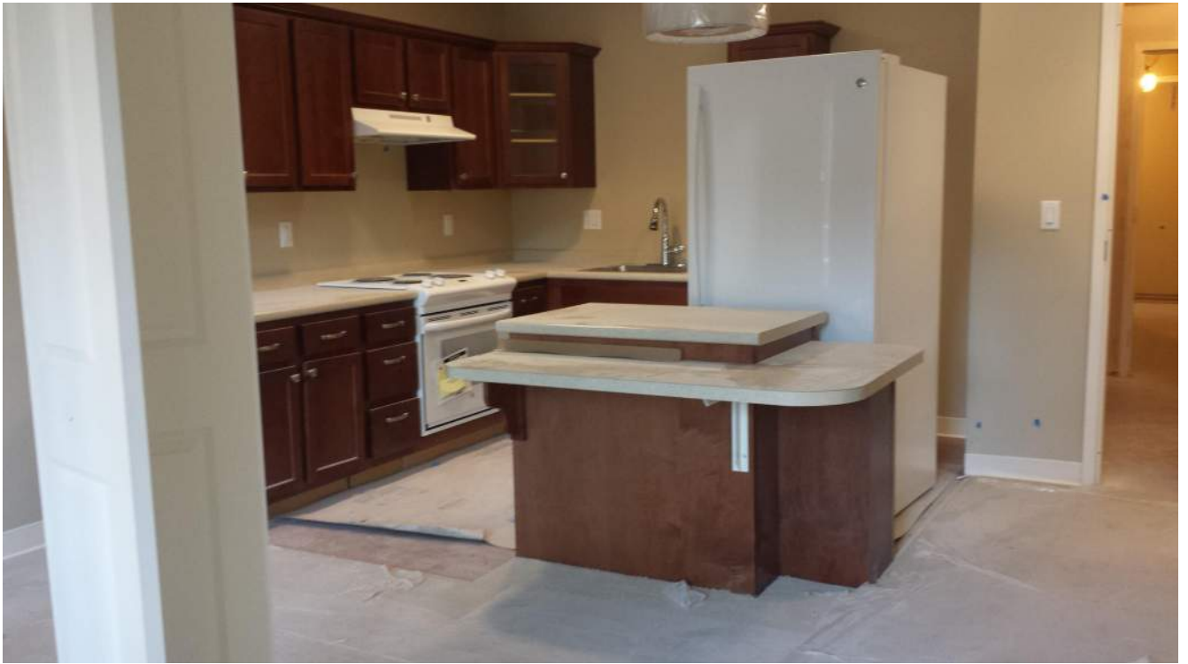
Levels 1 & 2 Typical Unit progress (Unit 1105 shown).
