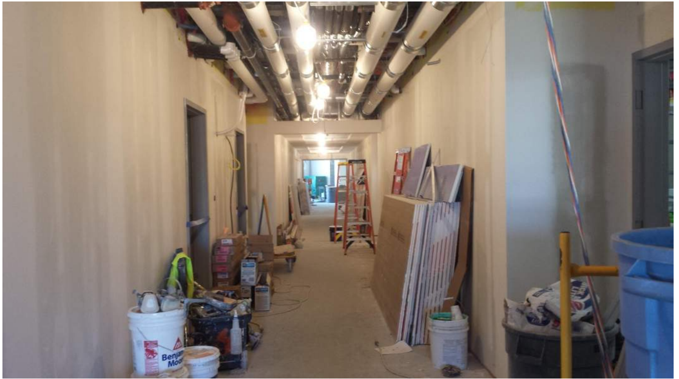
Level 1 New Construction West Wing
