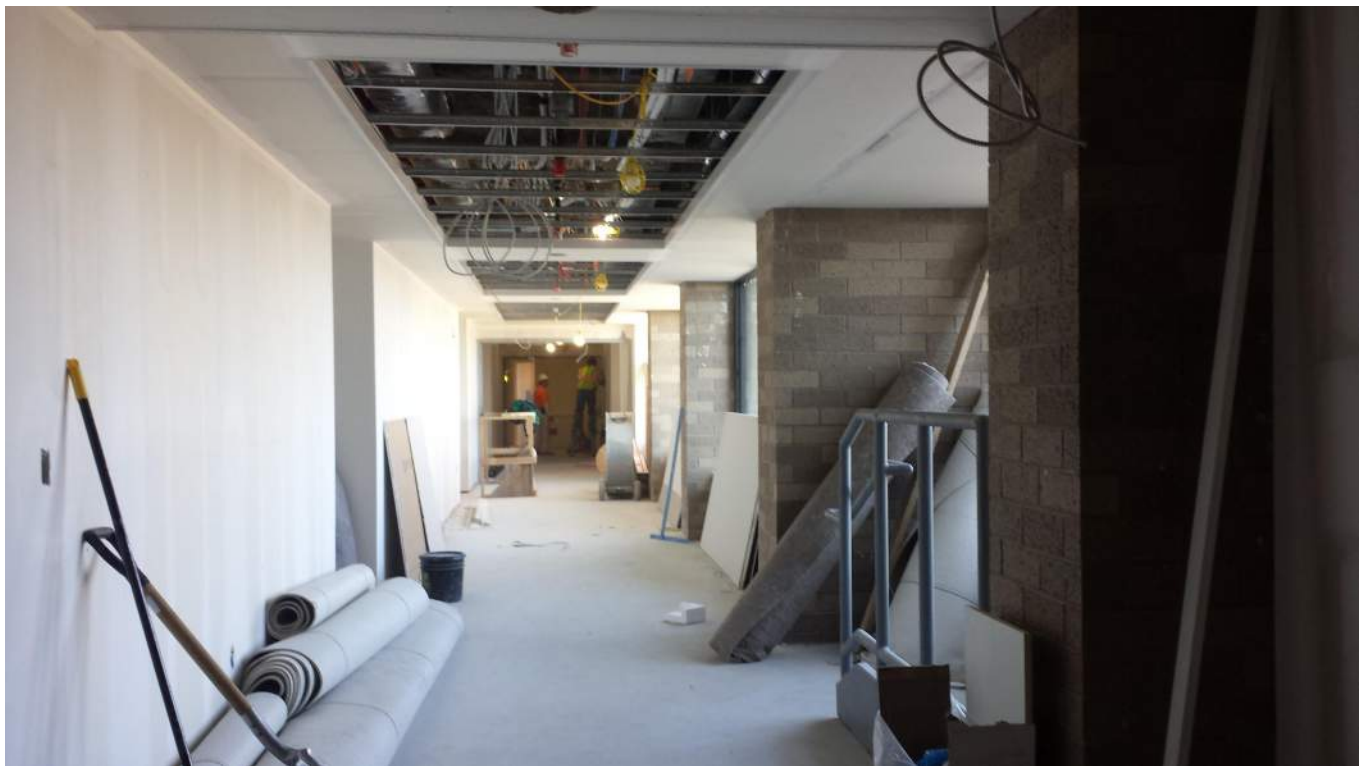
Level 5 New Construction East Wing
