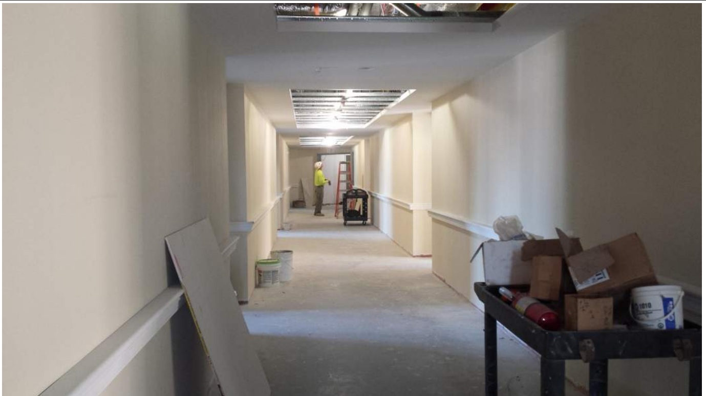
Level 3 New Construction East Wing
