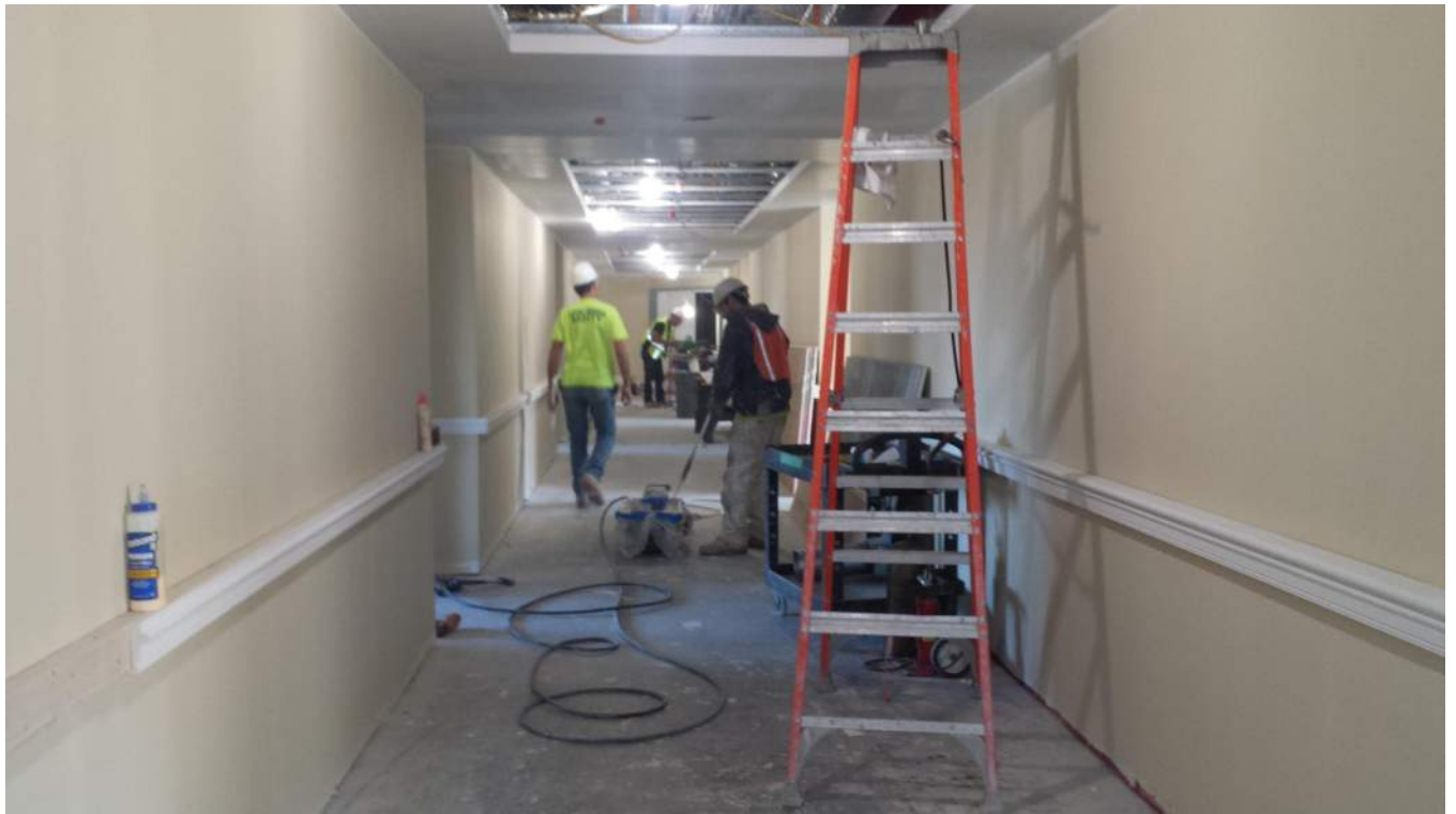
Level 5 New Construction West Wing
