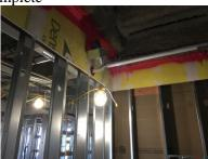
• Firestopping not consistent for heating pipes in exterior walls.
