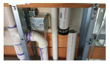
5. <u>Valve box drains still not protected</u>. Coordinate installation of washer, dryer, and AC drains.
