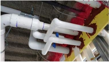
8. Fire proofing labeling is not consistent, many labels are missing.
