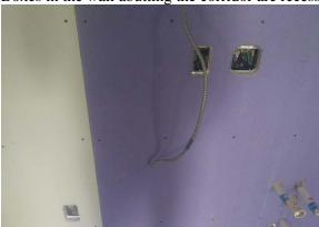
2. An air cap is visible at a cable penetration throught the wall abutting the corridor.
