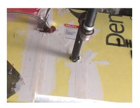
4. Repair damaged supply duct insulation.
