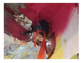
9. Cover washing machine standpipe during construction, some were covered, some not.
