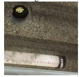
7. Seal holes in floor where not used for piping penetrations.
