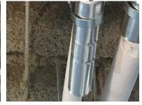
2. Adjust hangers so that piping is supported, and does not have any peaks or valleys in horizontal span and runs straight in vertical positions.
