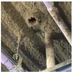
8. Seal supply duct insulation at fire rated wall.
