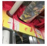
9. Verify fire caulking completely seals pipe penetrations.
