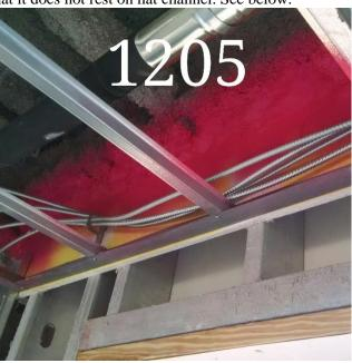
3. Fire caulk all penetrations through rated assemblies; re-apply when temporary wiring is removed. See below.
