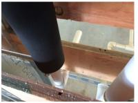
Complete firestopping, Seal large holes in gyp board where firestopping is required.
