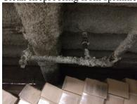
Provide cover/protection for plumbing fixtures, ductwork and piping during contruction.
