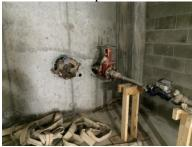
Piping in the Garage has been installed to maximize headroom, utilizing the precut holes in the beams. The vertical drops may be vulnerable to damage depending on where the parking areas are located.
