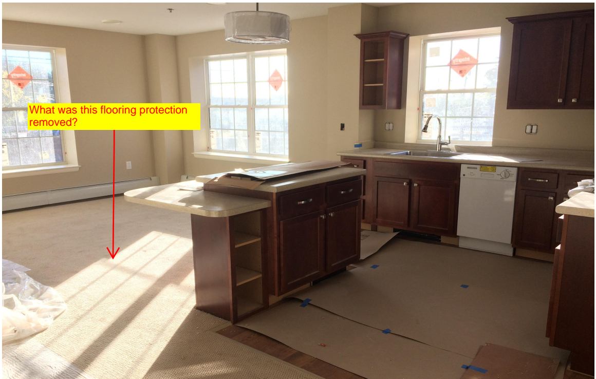
Corner Unit - Level 1 (Unit 1112)
