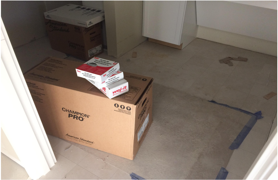
Flooring protection in typical bathroom
