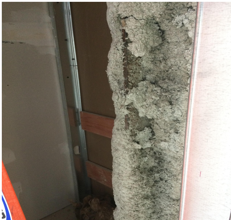
Steel column in Group Room 4004. Reference Item #22.5
