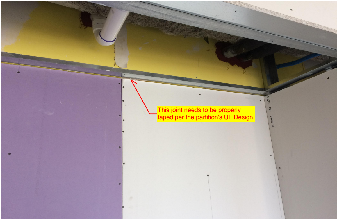
Group Room (4004) wall between group room and toilet rooms. Reference Item #22.5
