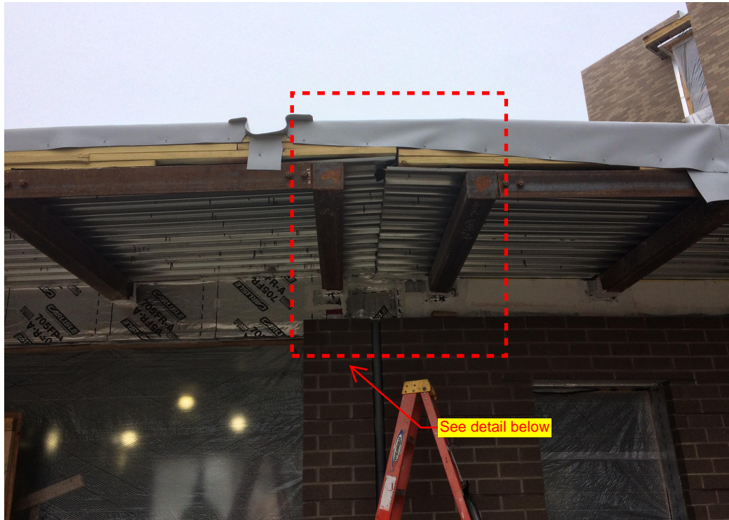
Canopy Expansion Joint - Reference Item 21.3
