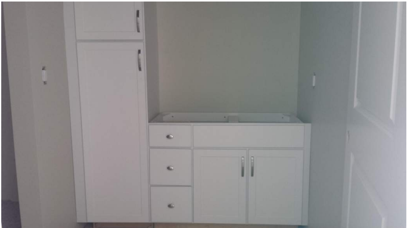
Typical Resident Bathroom casework progress, Levels 1-3 (Unit 1212 Shown)
