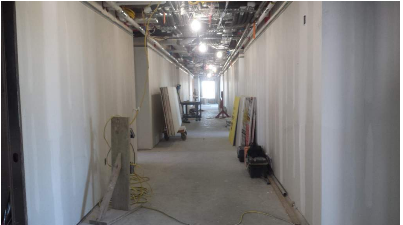
Level 5 West Wing
