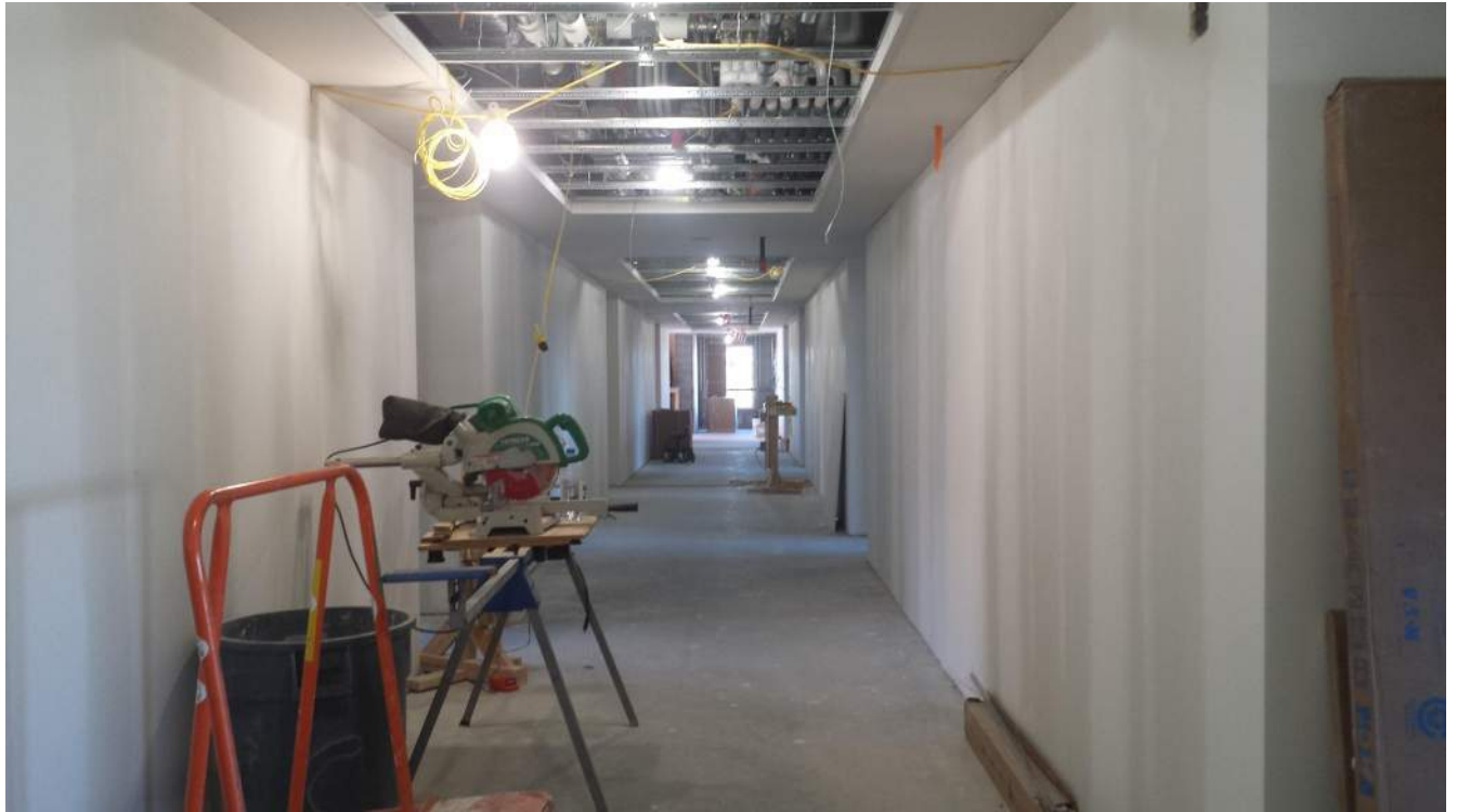
Level 4 West Wing
