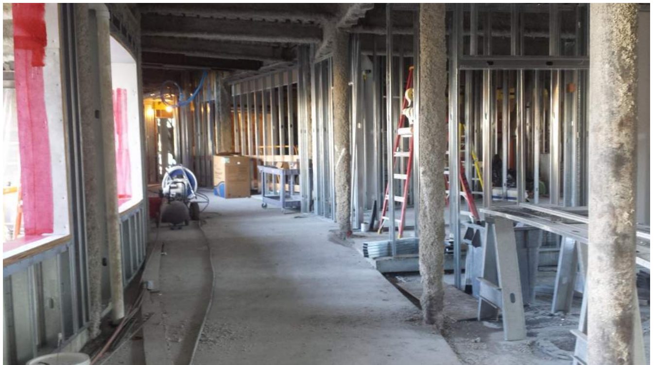
Connector from ramp/activity room
