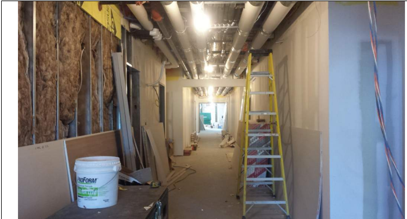
Level 1 West Wing
