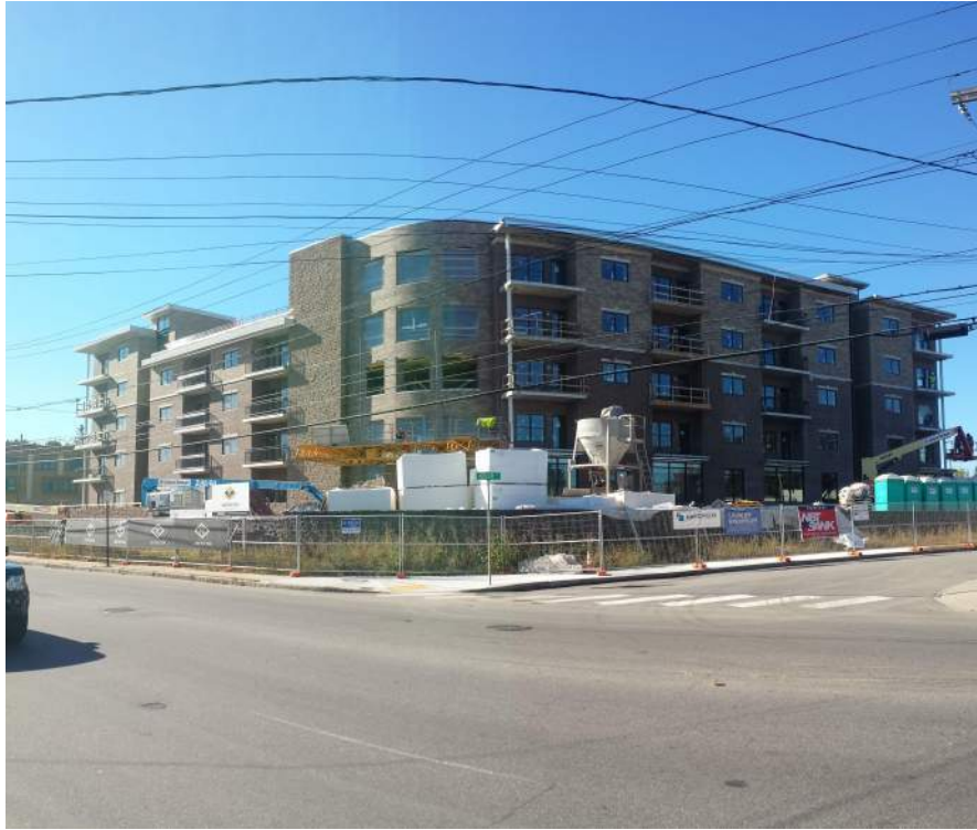
New Tower Construction from Forest Ave. at Arbor Street
