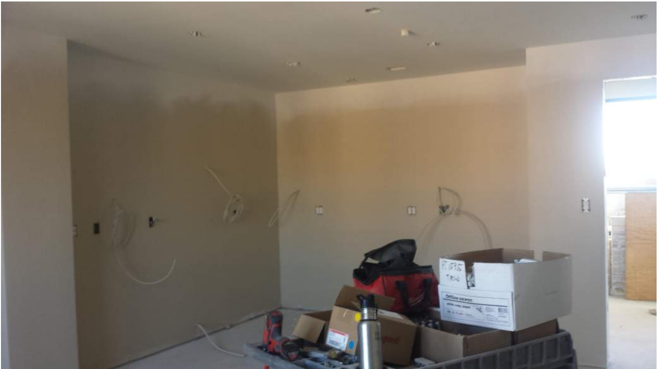
Typical Resident unit progress level 5 (unit 1507 shown).
