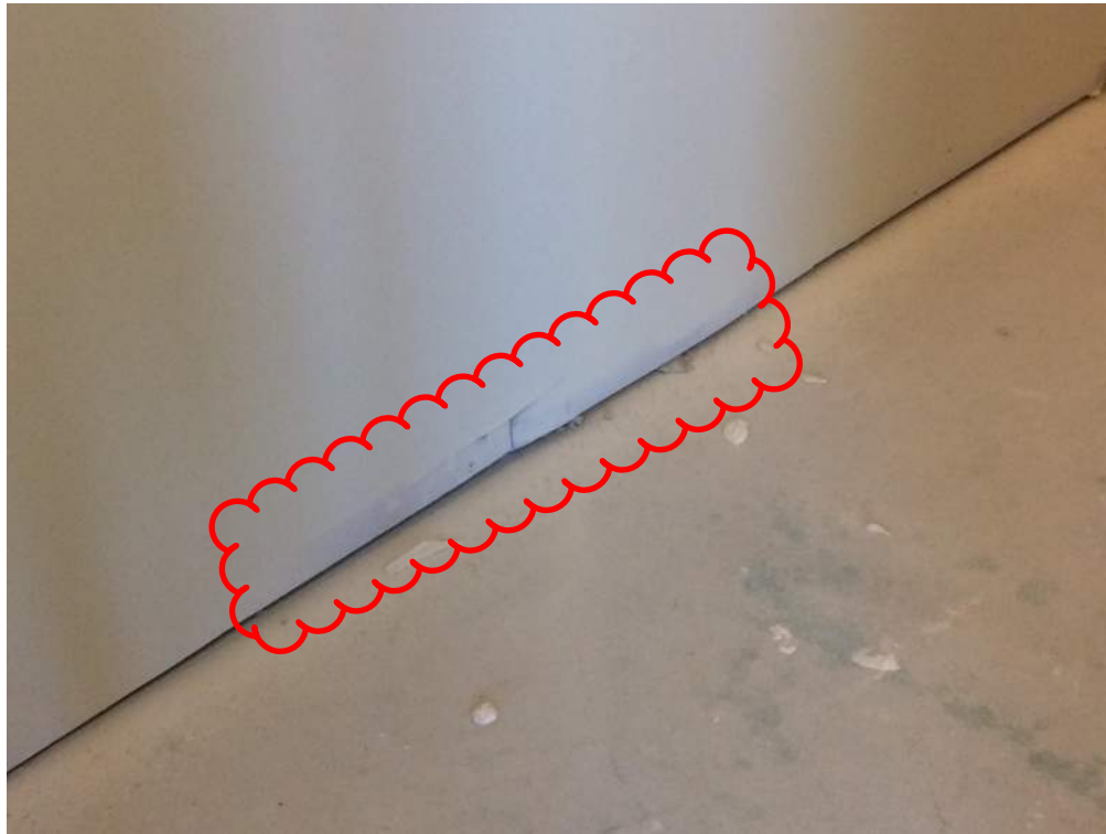
GWB Base at floor slab. See Note 20.08
