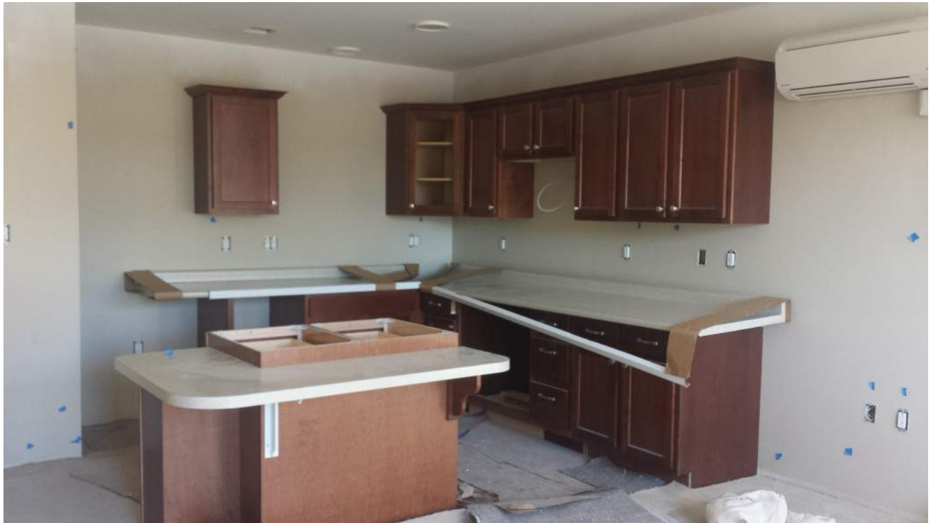
Typical Resident Kitchen casework progress, Levels 1-3 (Unit 1110 Shown)
