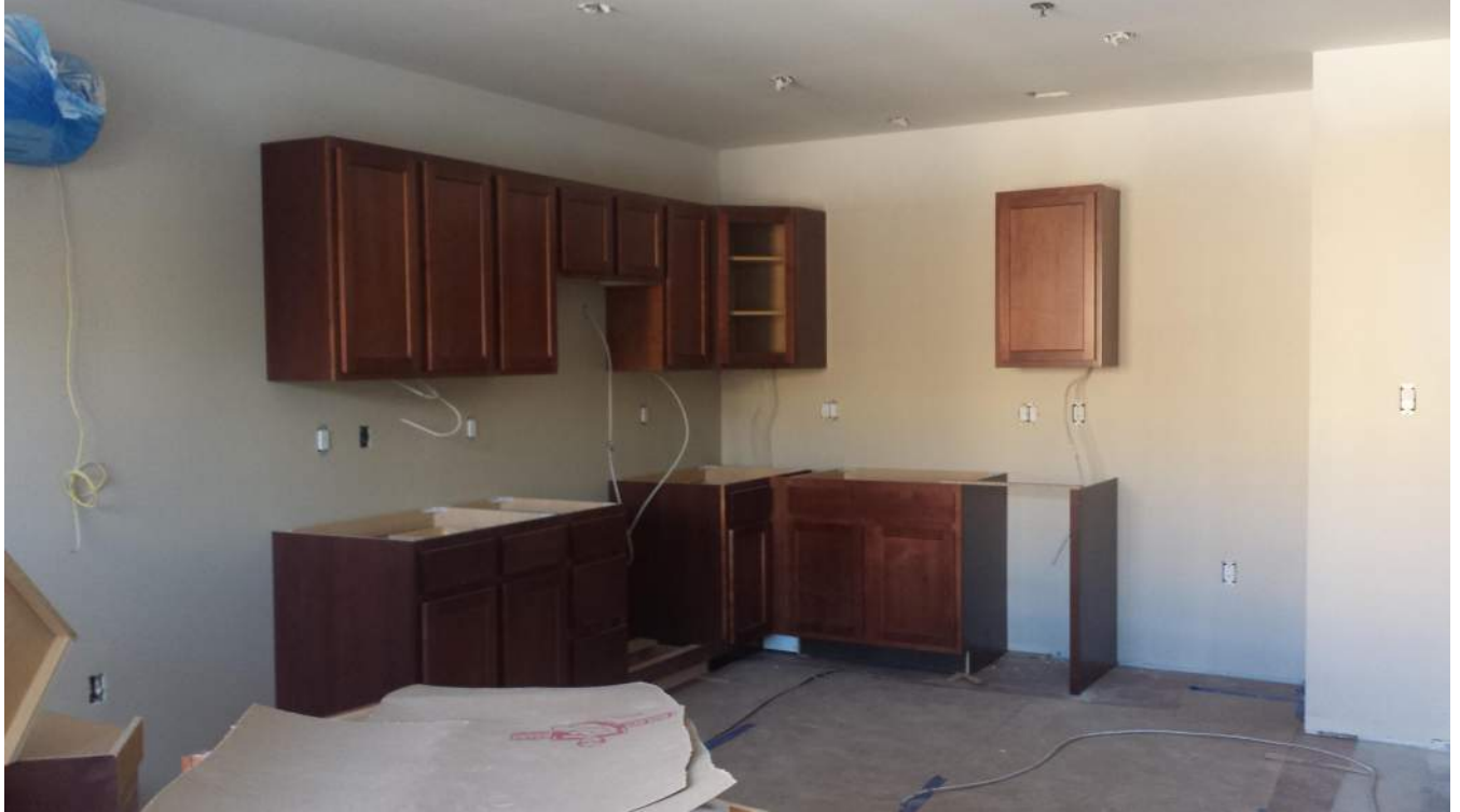
Typical Resident Kitchen casework progress level 4 (unit 1409 shown)
