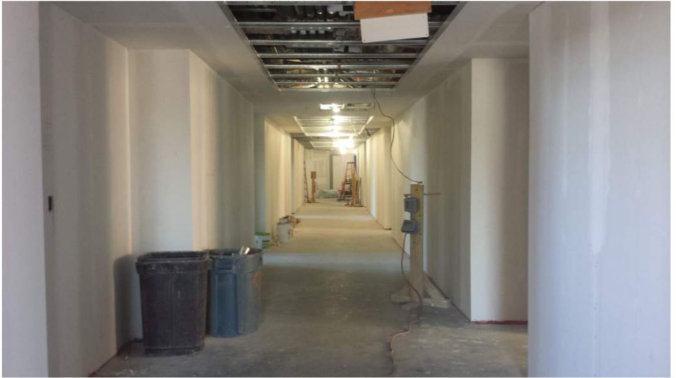
Level 3 West Wing
