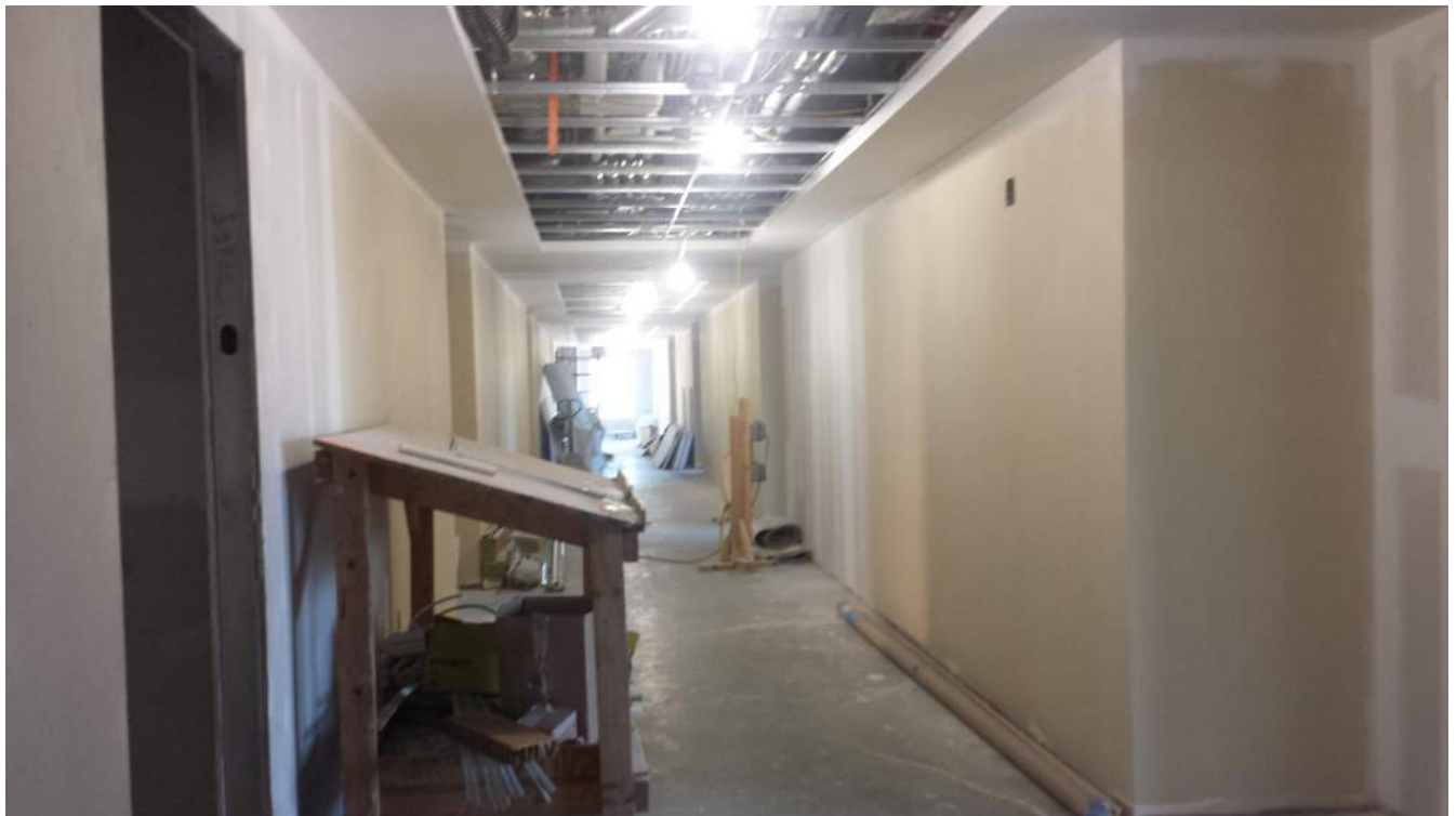
Level 2 West Wing
